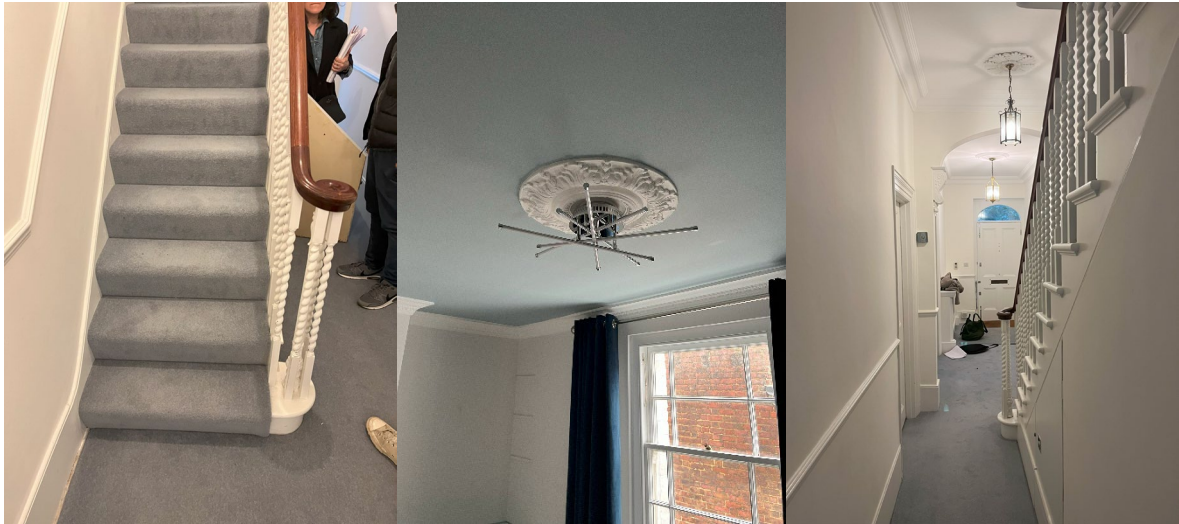
Figure 7: Internal photographs highlighting the current condition of the property and any existing period features
