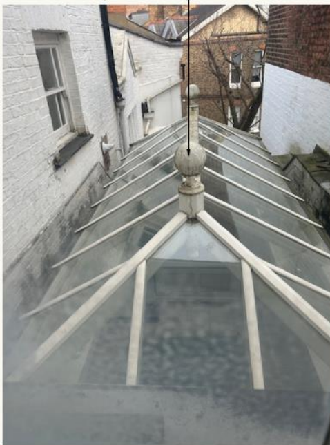
Non-original skylight above previous courtyard extension
