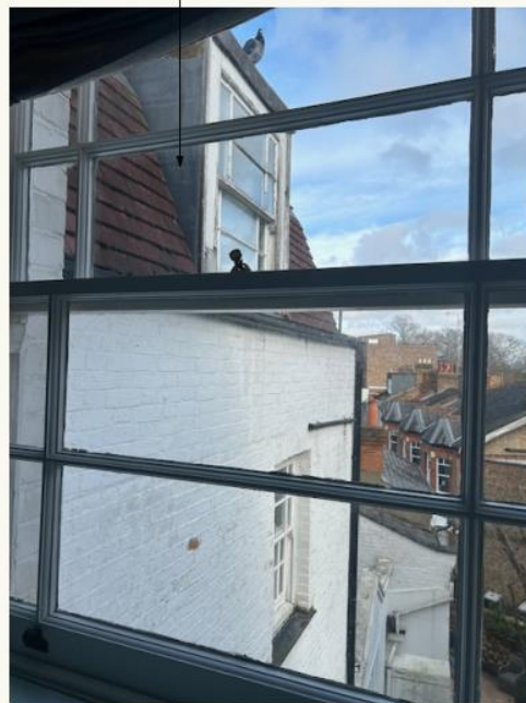
Non-original dormer window extension (existing)
