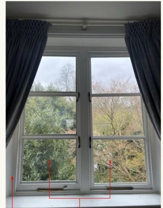
Original main frame, non original casement frames, non original glass.
