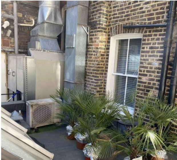
Photograph 3 – Rear of 10 Charlotte Street and rear of 8 Charlotte Street.
