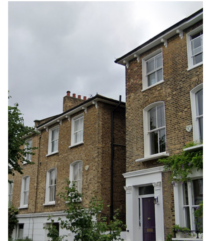
View From street showing wide eaves and shallow roof formation
