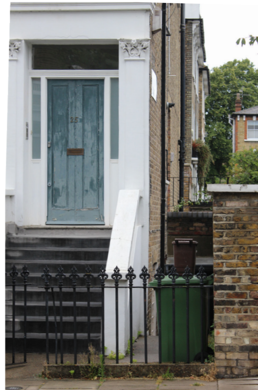
Decorative metal railings, finished in black and white plaster detailing
