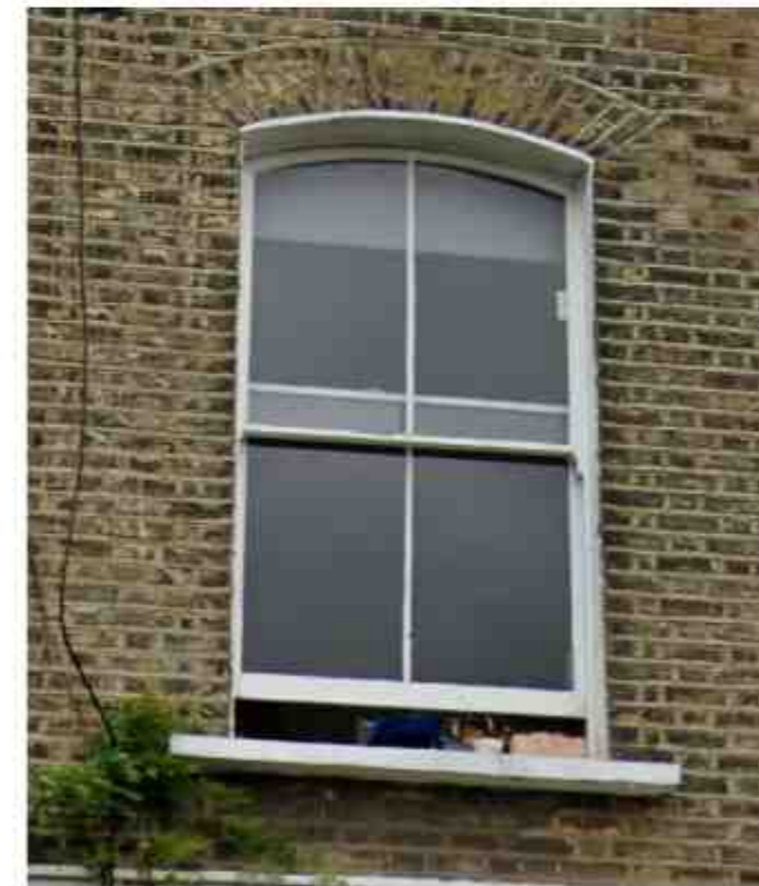
White Painted timber sash windows with white plaster detailing to sill. Soldier course brickwork lintel
