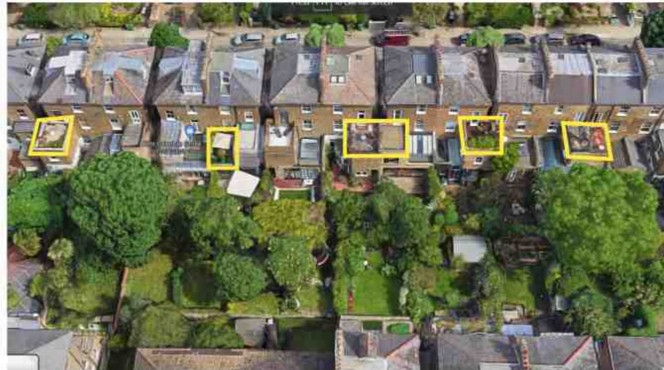
Patshull Road roof terrace
