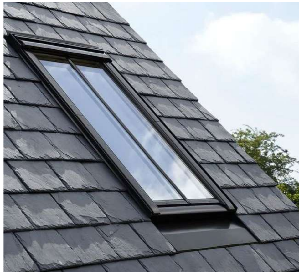
FIGURE 13: CONSERVATION ROOF LIGHT IN-SITU
