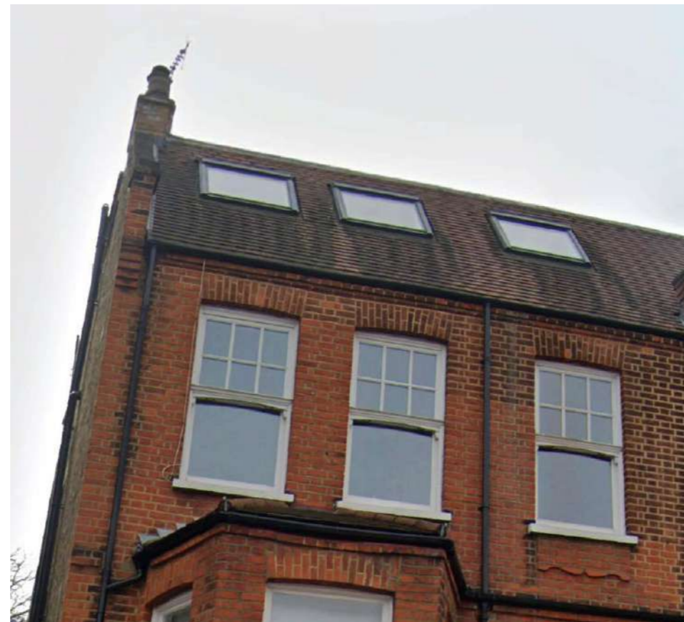
FIGURE 11: CONSERVATION ROOFLIGHTS USED AT 67 GREENCROFT GARDENS
