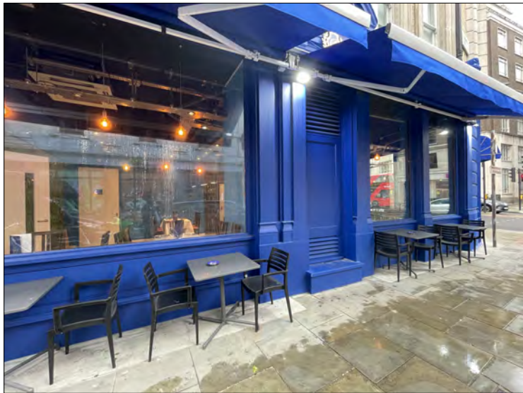
EXISTING SITE PICTURES
