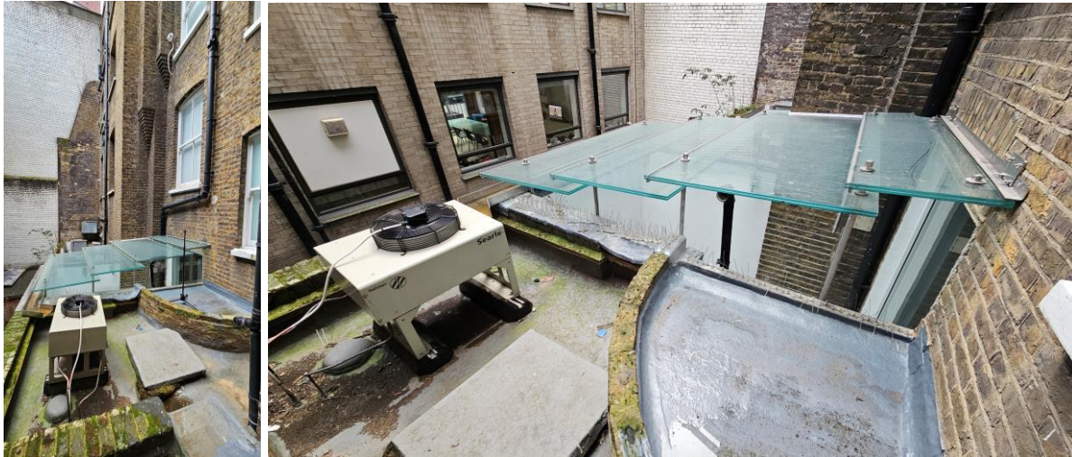
Picture 1: Residential NSR and external cellar cooling unit locations
