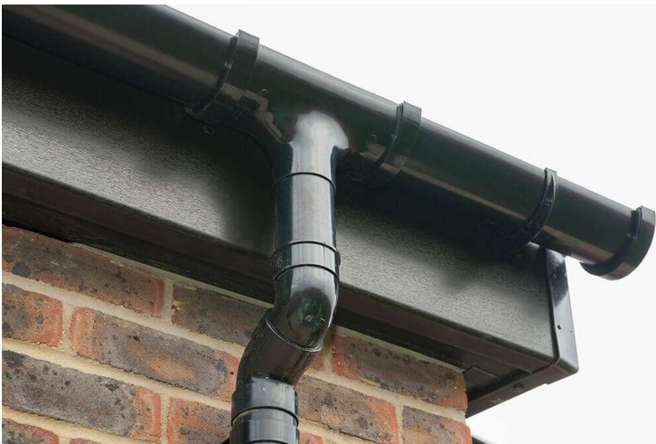
Image 05 – Black Upvc rainwater goods
