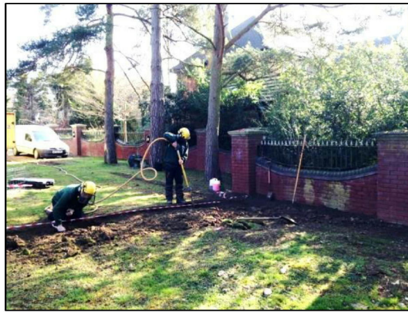
Figure 3: Image of Bartlett Tree Experts Using Air Spade within Root Protection Area
