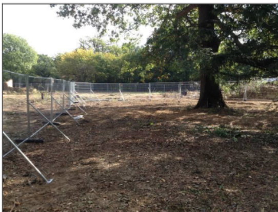
On site examples of appropriate tree protection fencing installed as recommended within BS5837
