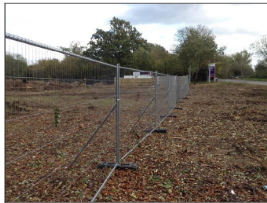
On site examples of appropriate tree protection fencing installed as recommended within BS5837
