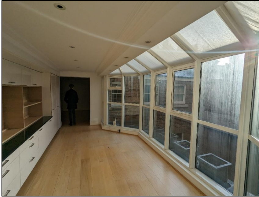
Figure 4.4: Ground floor extension, added in the 1990s, with conservatory style PVC framed windows
