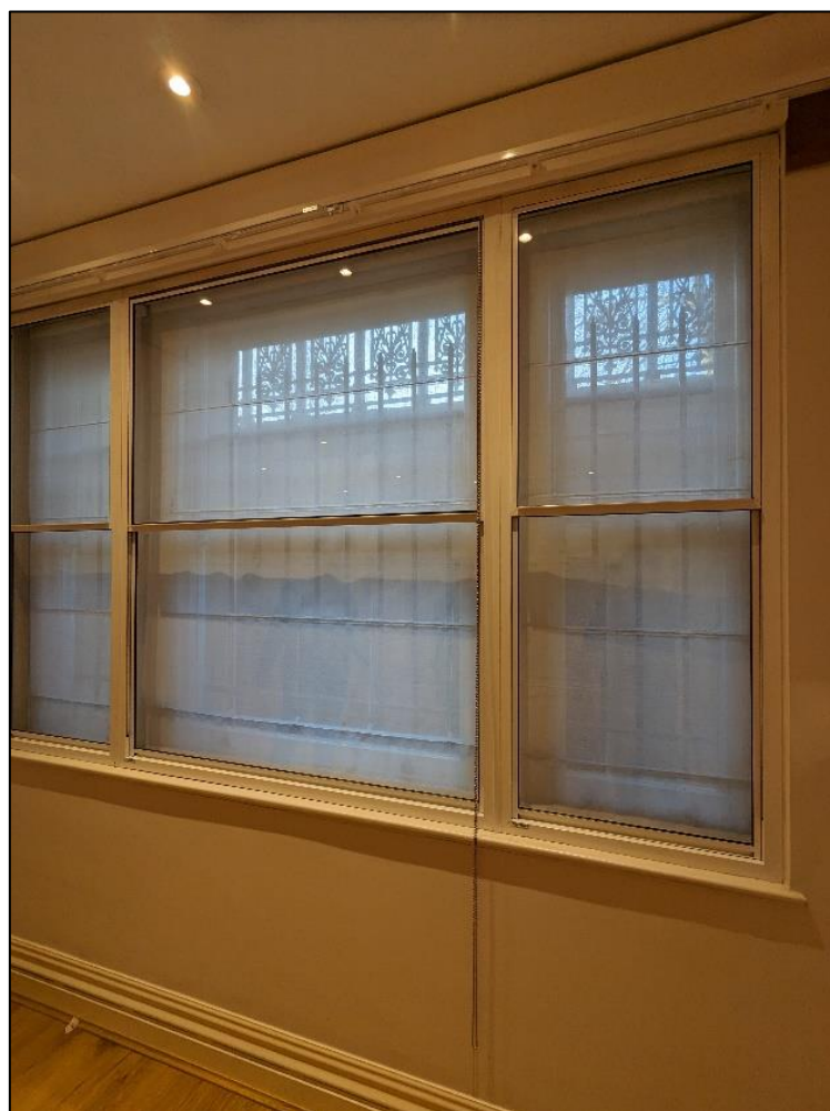
Figure 4.7: Altered skirting, modern fit-out and modern secondary glazing found in basement level front room
