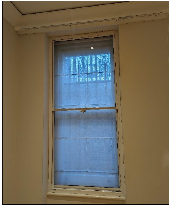
Figure 4.8: Secondary glazing with poor visual quality in the basement level front room
