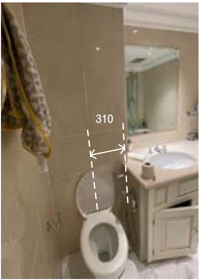
Bathroom 1 - below minimum standard toilet to wall and sink distances in shared bathroom
