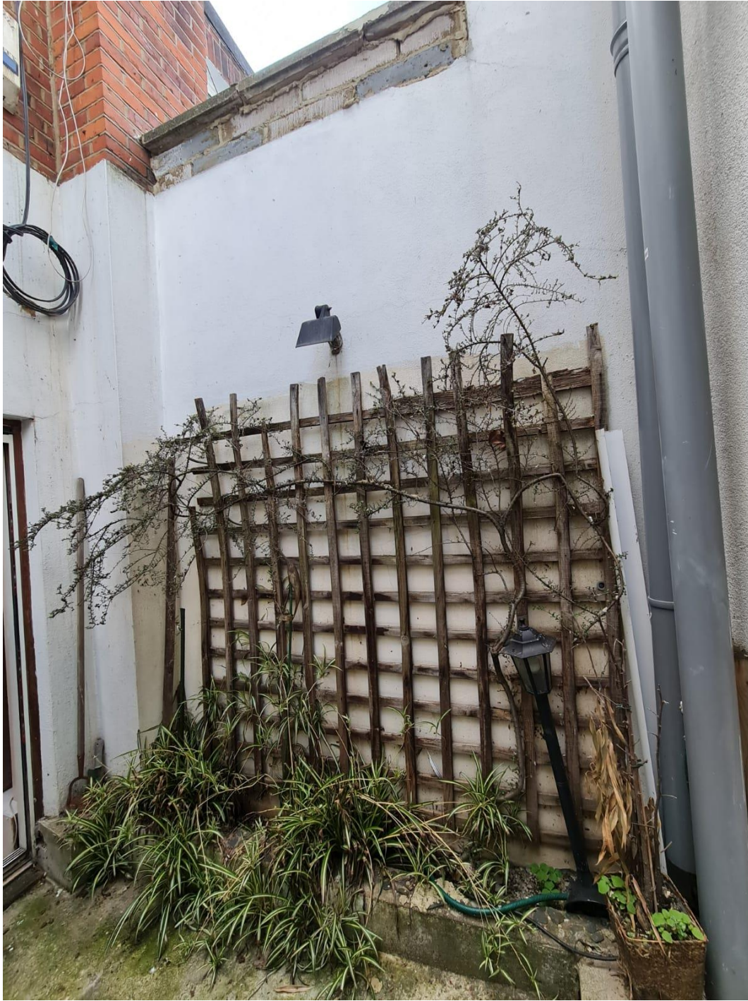
Rear courtyard looking north
