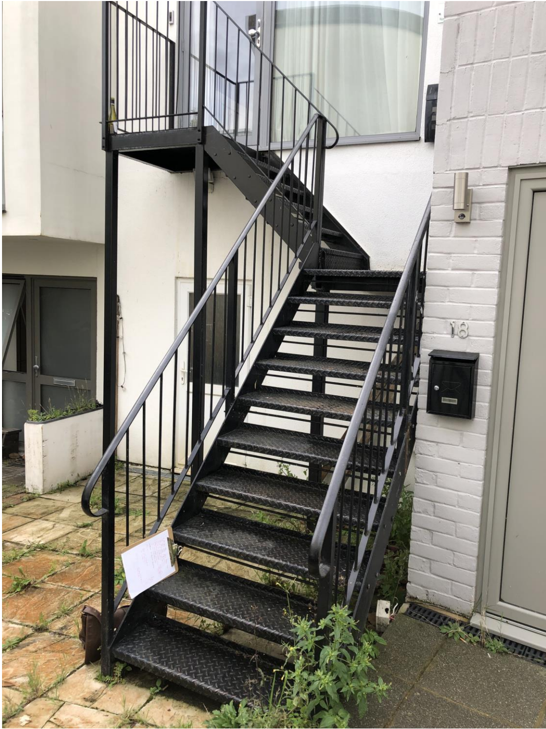
Rear access staircase
