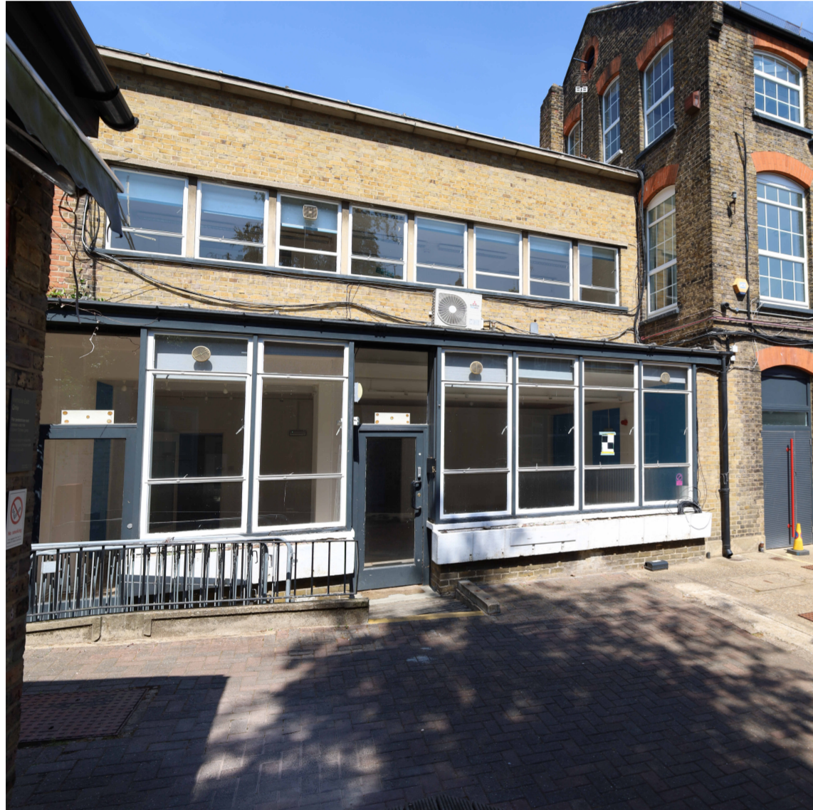
PHOTOGRAPH AS EXISTING
