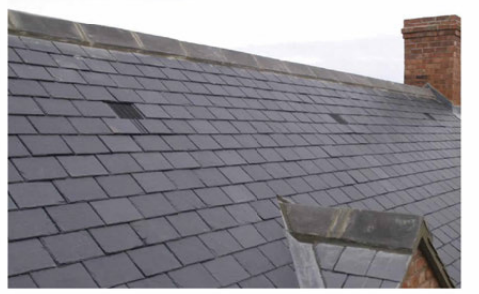
In-Line Roof Vent System Roof vents indicated light purple to existing principal roofs contoured to match tile profile to M. Eng details
