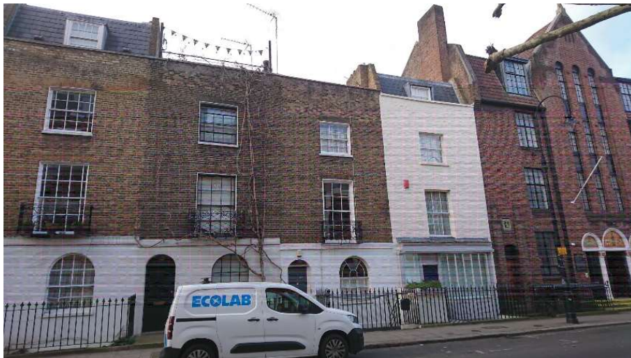
Photograph 2: Arlington Road Elevation Showing 155-161 (No 161 is white painted building)
