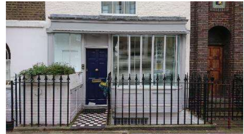
Figure 8: No161 Front ground floor shop-front.
