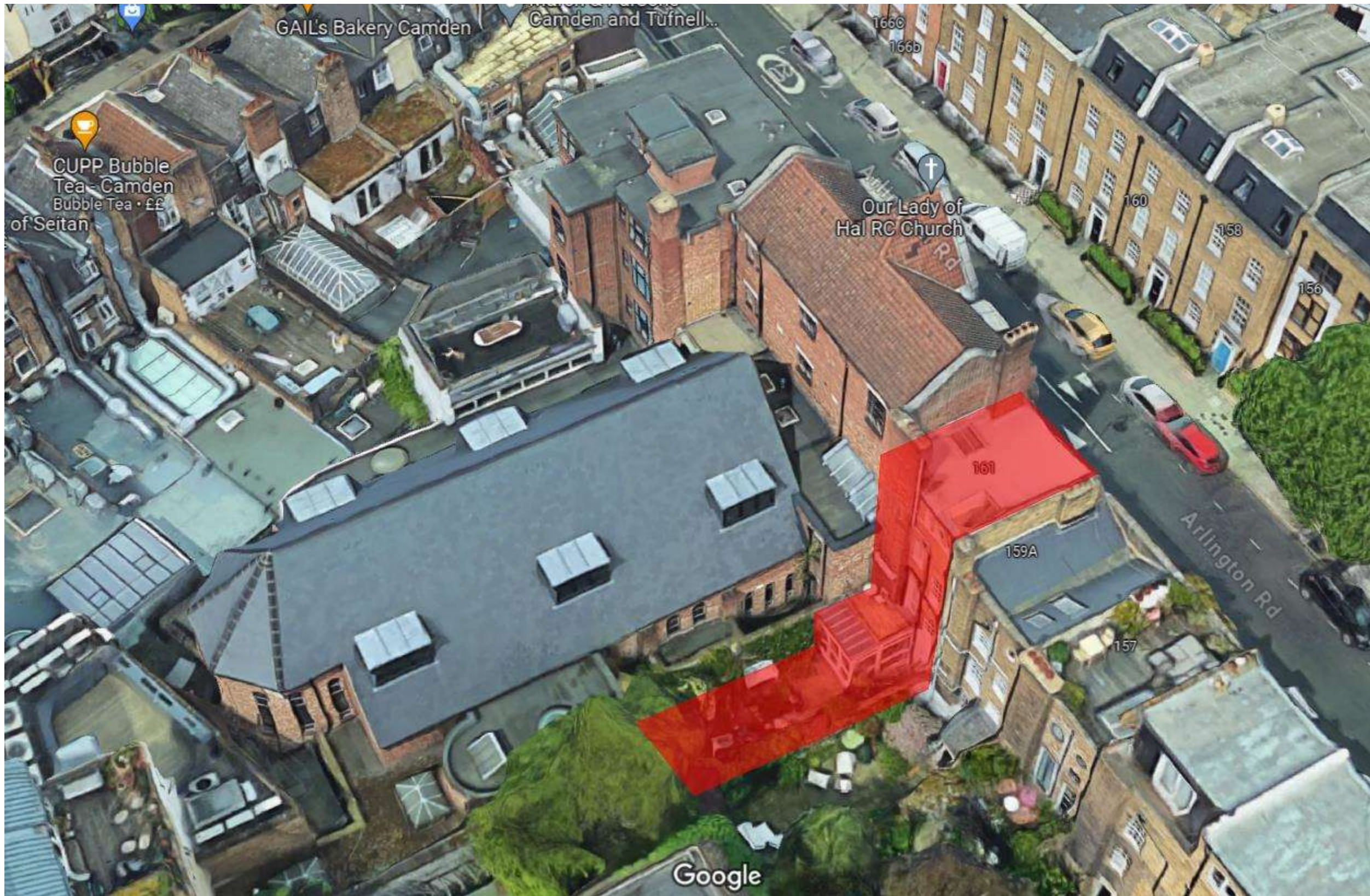
Fig 5: View of 161 Arlington Road from Rear Showing Neighboring Buildings
