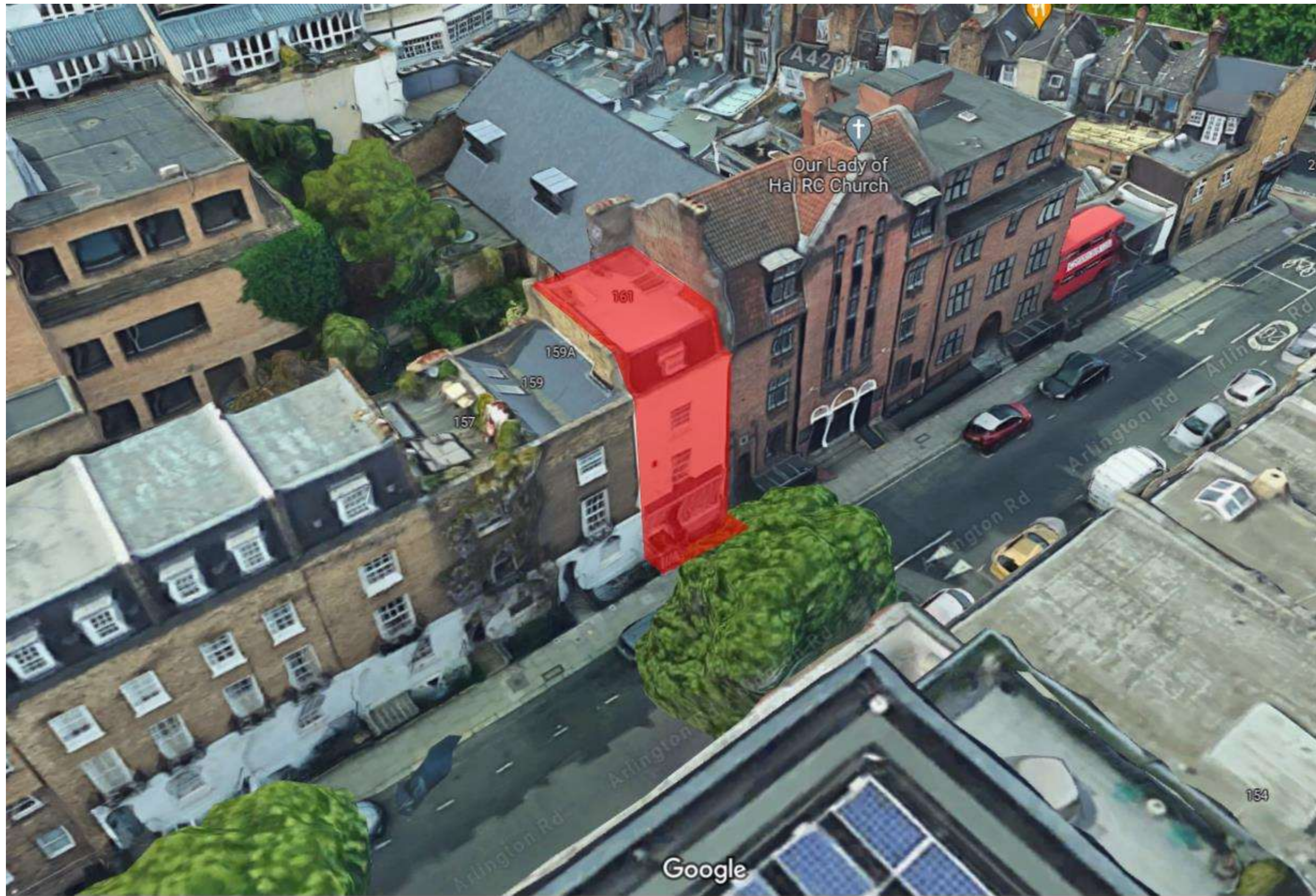
Fig 4: View of 161 Arlington Road from Front Showing Neighboring Buildings
