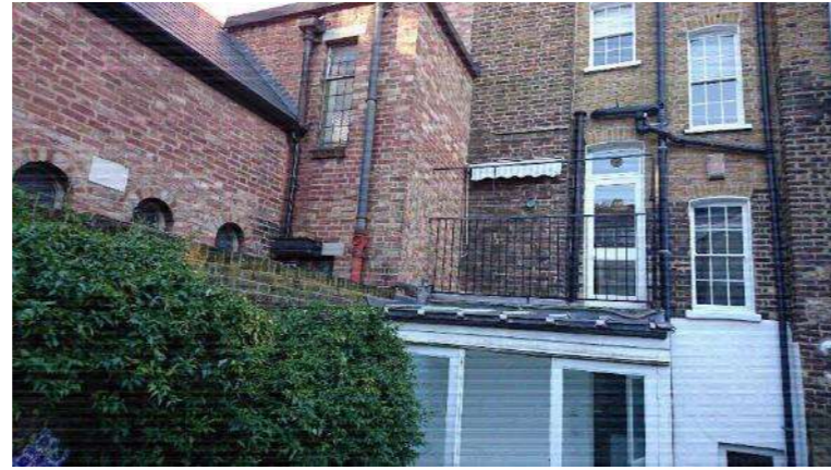
Photograph 7: Rear Elevation looking North
