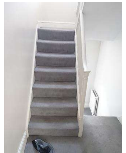
Main stair at ground
