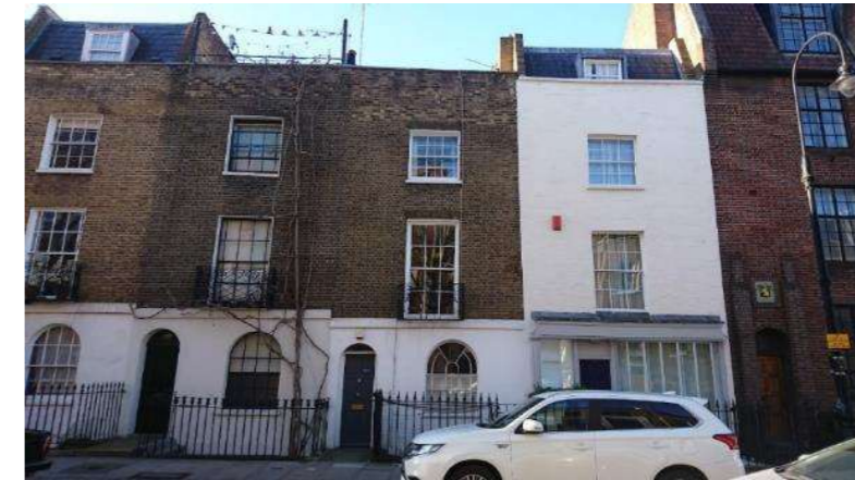
Figure 1: Street view of 155-161 Arlington Road (No161 is white building on right)
