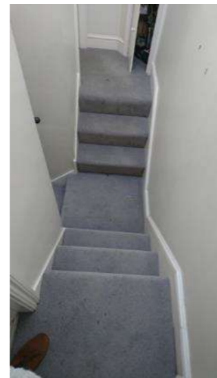
Photograph 42: Top section stair second to third
