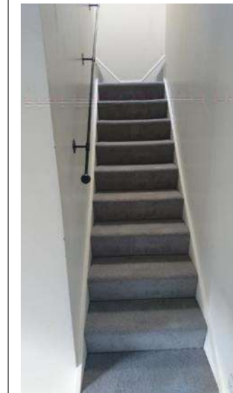
Photograph 41: Stair second to third
