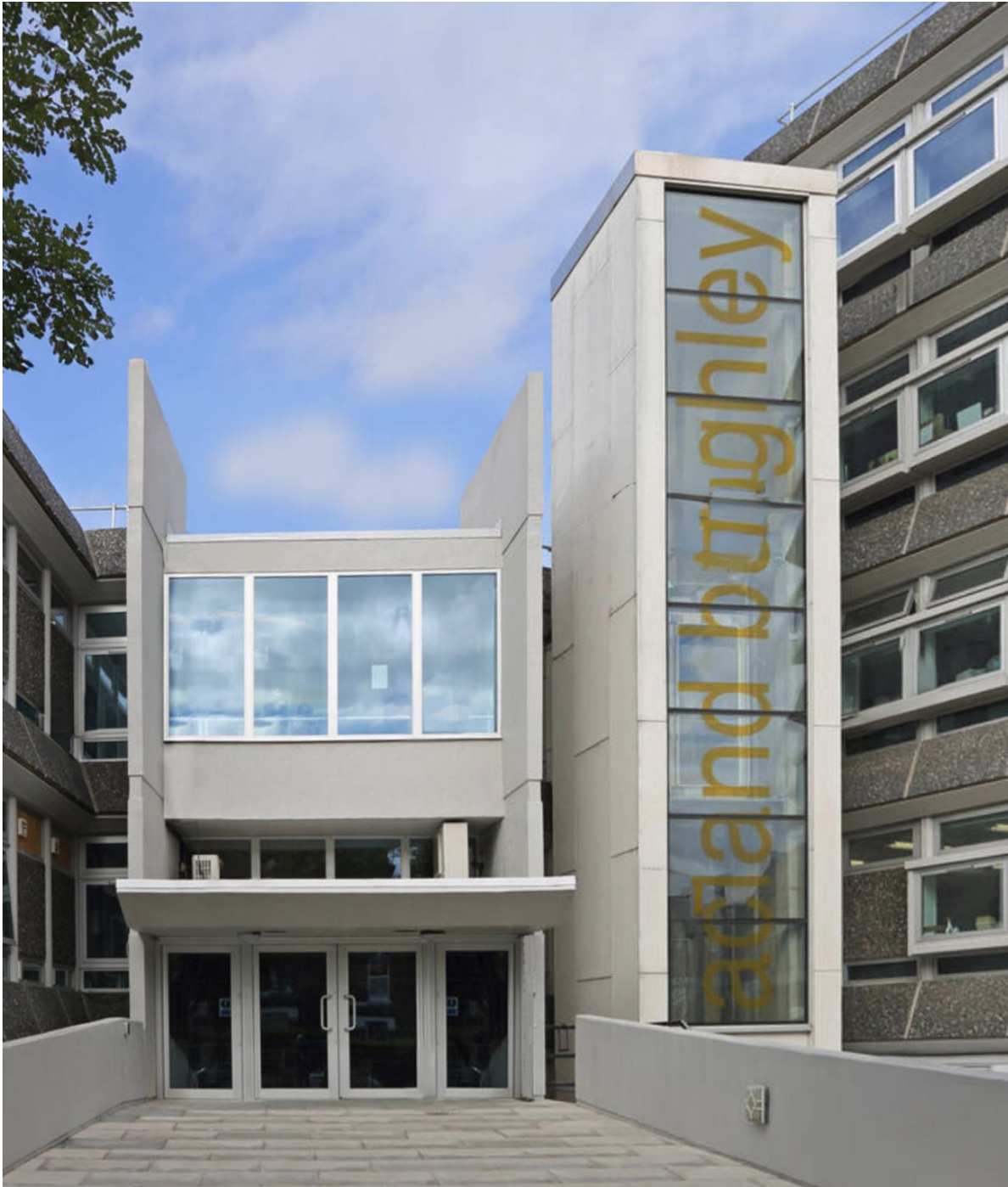
EXISTING ENTRANCE DOOR
