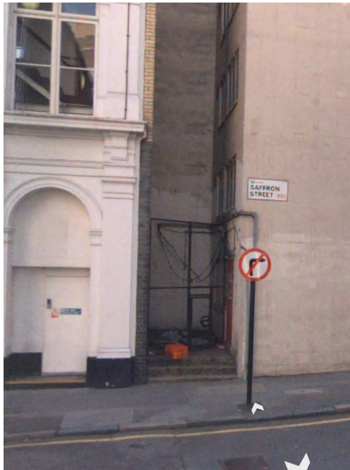
Existing condition showing accumulation of rubbish
