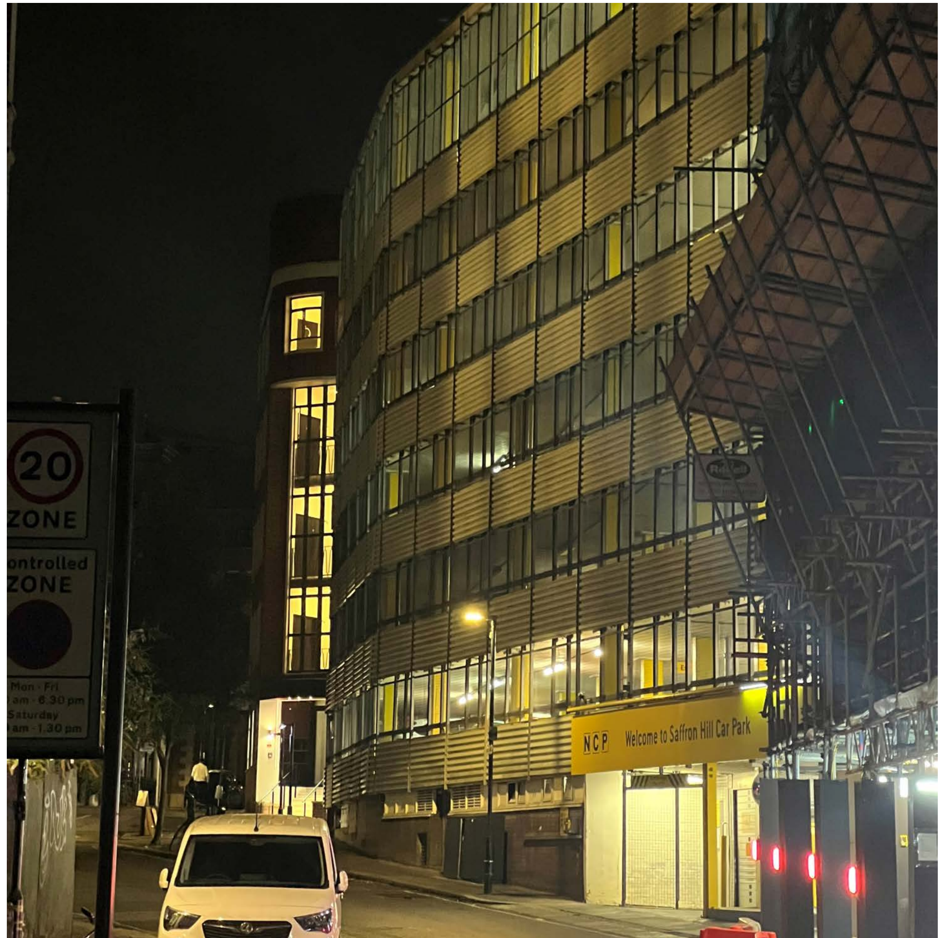
Existing Car Park
