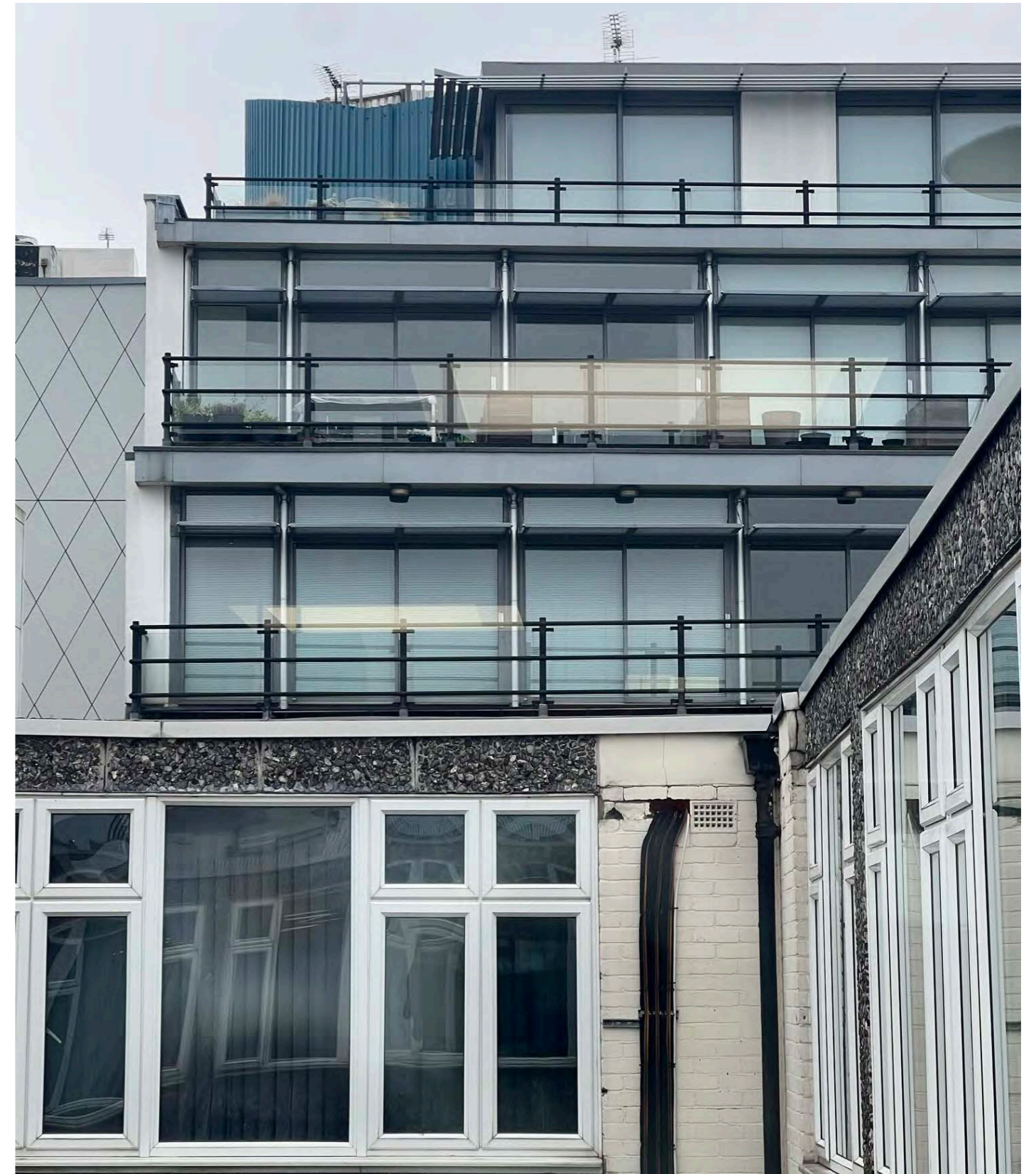
View from the NCP offices towards Ziggurat, level 08.
