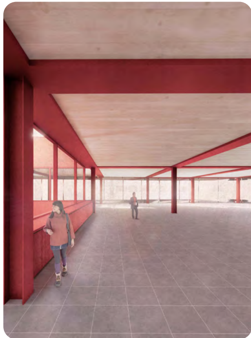
Precast Delta Beams with CLT Infills
