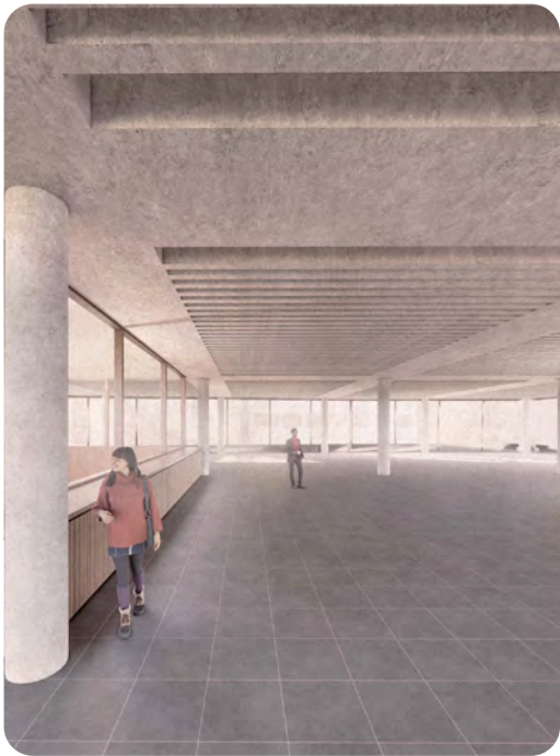
RC Frame with Ribbed Slab
