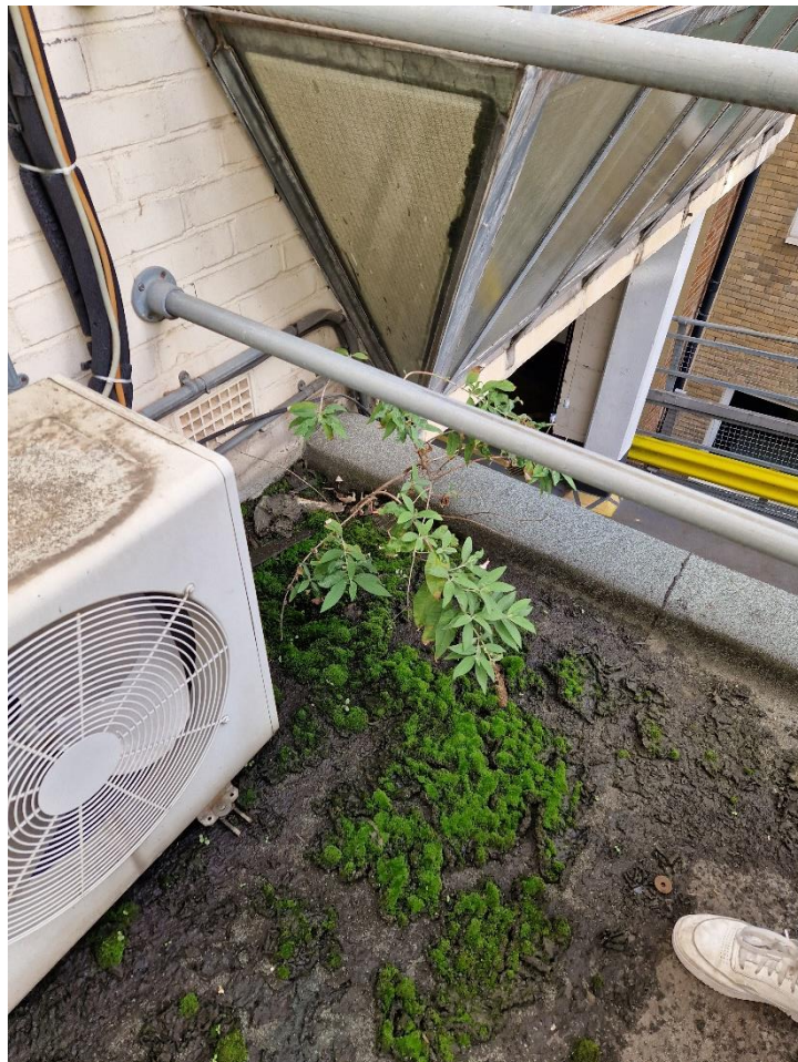
Photograph 4: Butterfly-bush (INNS1, Figure 1) and moss growing on the roof of building B1
