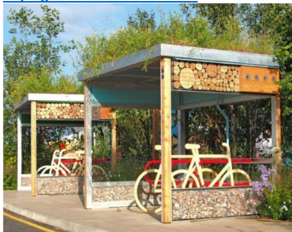
Figure 1. Example of green roofed cycle store http://greenroofshelters.co.uk/
