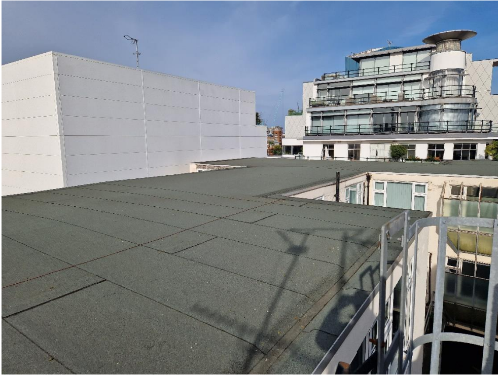
Photograph 5: Office building with felt roof and metal capping
