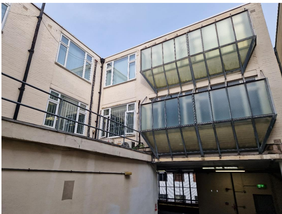
Photograph 2: Two-storey office extension on building B1
