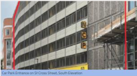
Car Park Entrance on St. Cross Street, South Elevation
