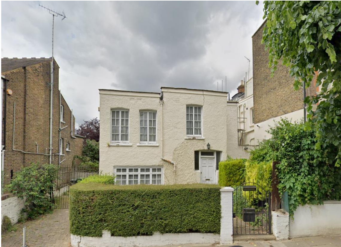
The Cottage, Hilltop Road – street elevation
