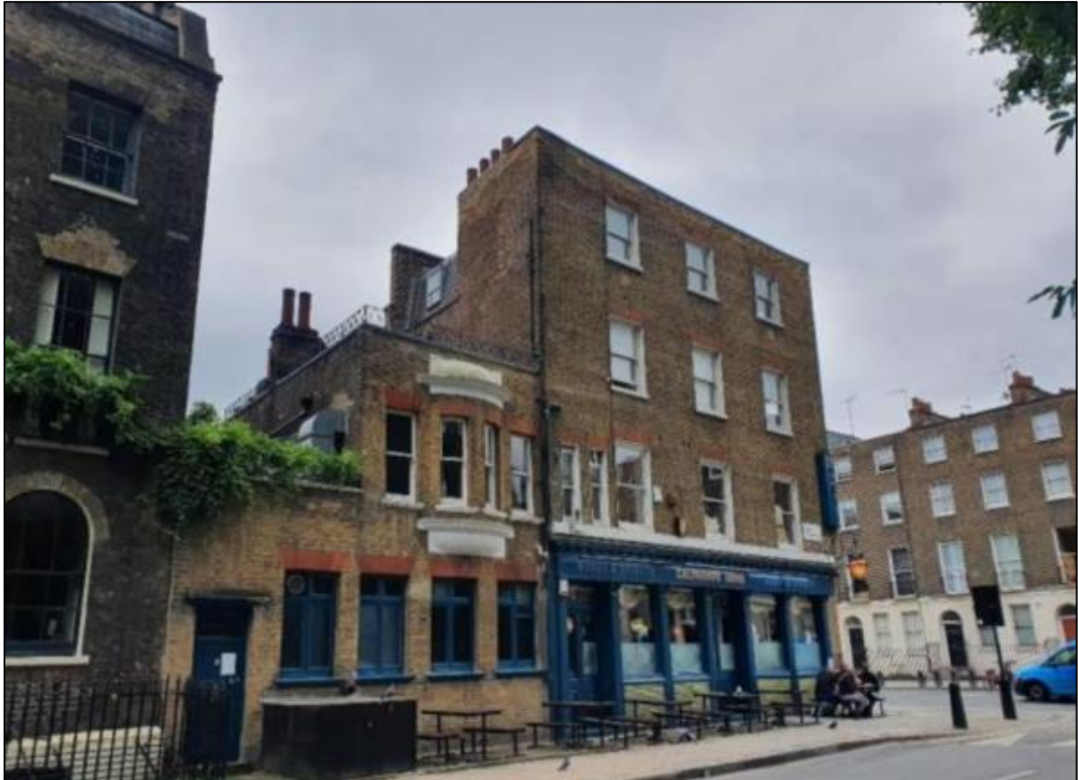
Fig 1. Existing Wren Street (north) elevation
