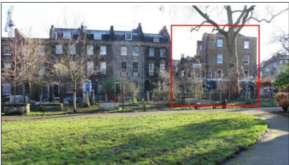
Fig 2. Existing Wren Street (north) elevation when viewed from St Andrew's Gardens (locally listed)
