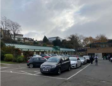
view of car park towards Giles Slaughter Wing
