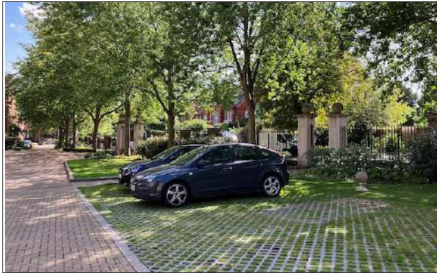
Existing Parking at UCS: reinforced grass
