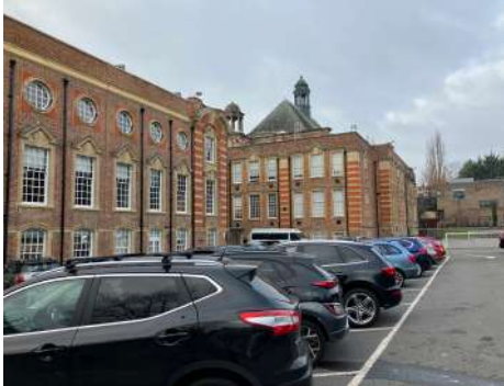
view of car park towards North Block
