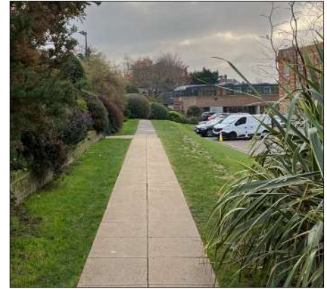
Existing Paving to be lifted & reused
