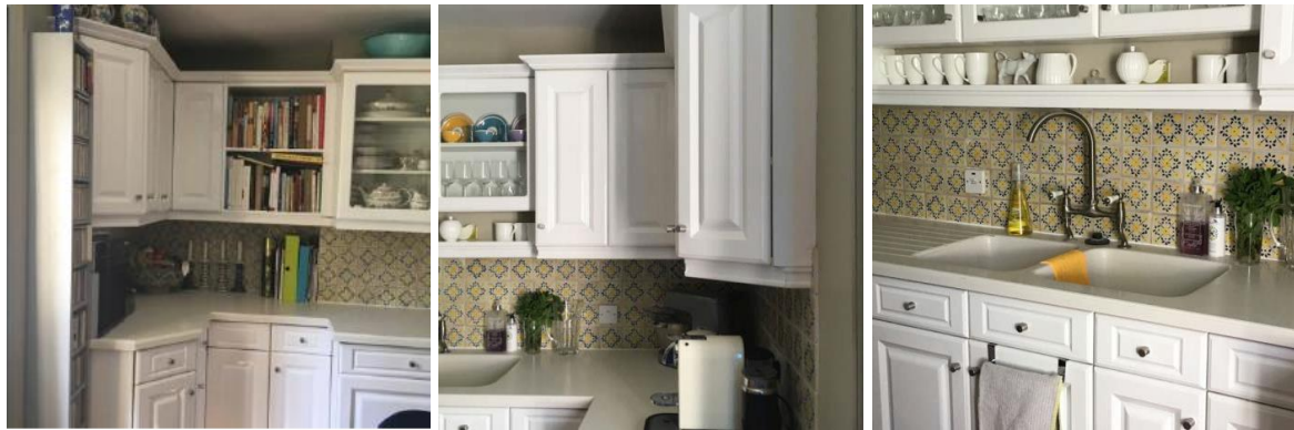
Figure 3: Existing kitchen units
