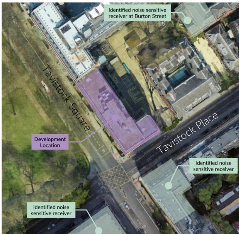
Figure 1: Site context showing the development location and nearby identified noise sensitive receptors.
