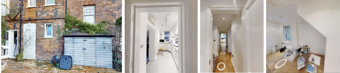
EXISTING SIDE ELEVATION / EXISTING KITCHEN (LOWER GF) / EXISTING CORRIDOR (LOWER GF) / EXISTING SW ROOM (LOWER GF)
