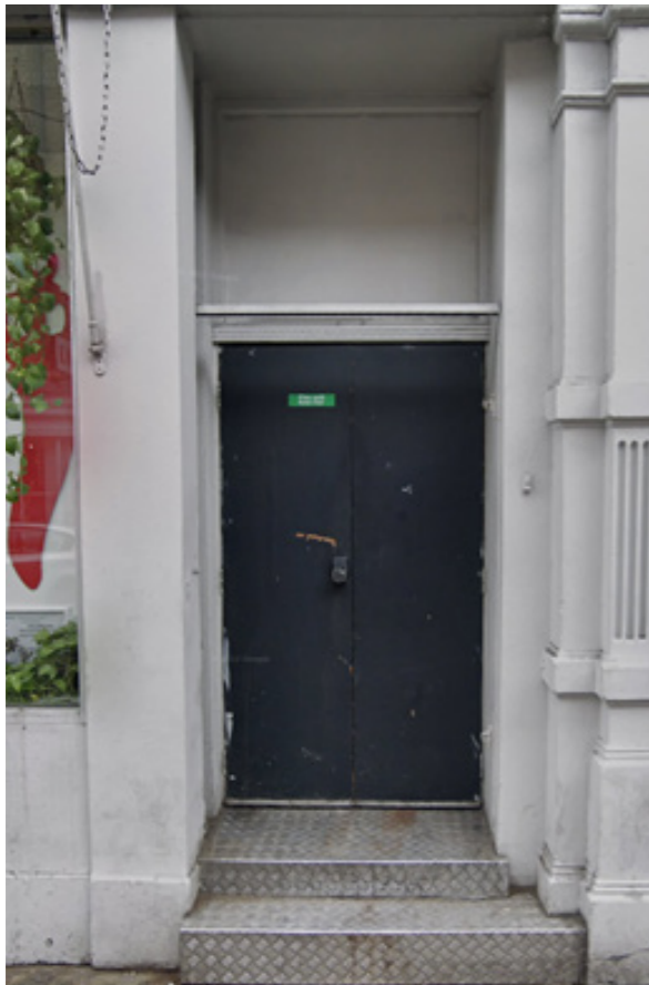
▲ Existing Monmouth Street Entrance
