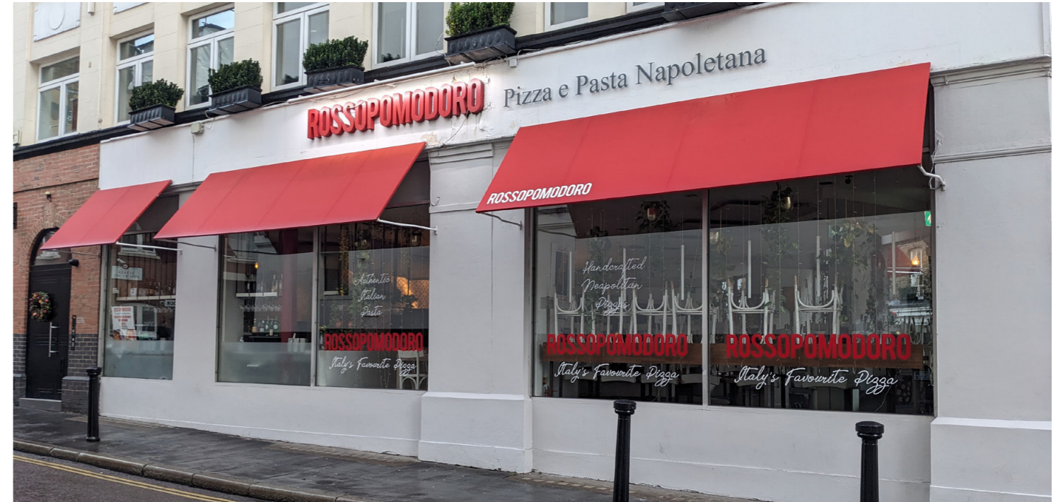
02 View of the site from Tower Street
