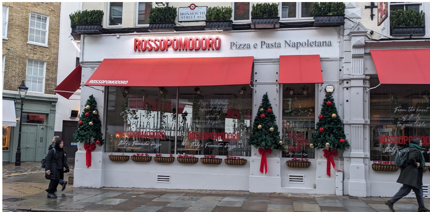
03 View of the site from Monmouth Street
