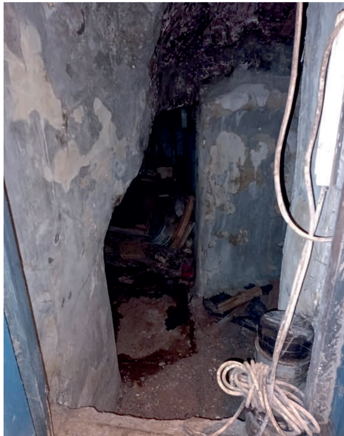
Fig 12 A vault in the basement's toilet (MOLA photograph 2023)
