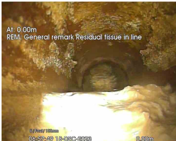
BR3X_e535855a-b95d-4030-aad8-14c0d10b1db9_20240108_121836_436.jpg, 00:00:09, 0.00 m General remark, Residual tissue in line
