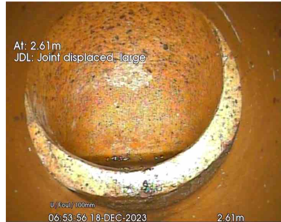
BR2X_e39a5c13-c1fe-4e56-b267-fdbcd2ab4d19_20240108_1 15759_634.jpg, 00:01:15, 2.61 m Joint displaced, large
