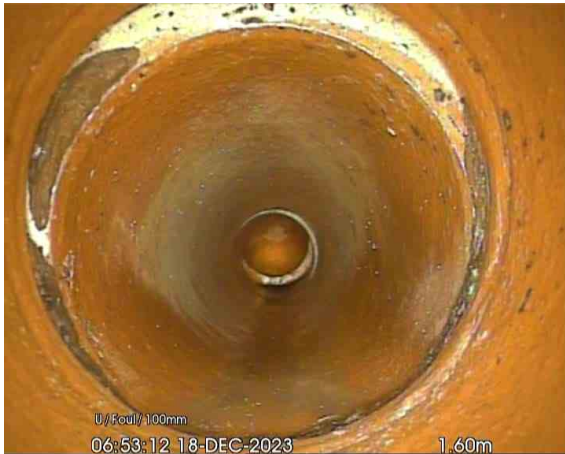
BR2X_f541e4ca-69e3-4271-a8e4-cf0b007e6738_20240108_1 14833_799.jpg, 00:00:47, 1.60 m Joint displaced, medium
