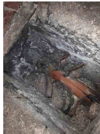
Unable to survey MH4 downstream due to seized rodding eye bung
