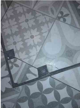
Manhole ouside female toilets cracked upon arrival (before lifitng)
