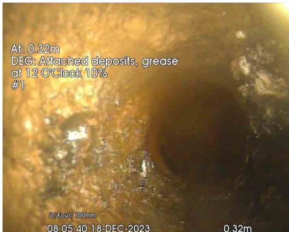
BR4X_cdec9da9-966c-43d6-b659-e4e94cae2322_20240108_131042_406.jpg, 00:00:25, 0.32 m Attached deposits, grease at 12 o'clock, 10% cross-sectional area loss, start
