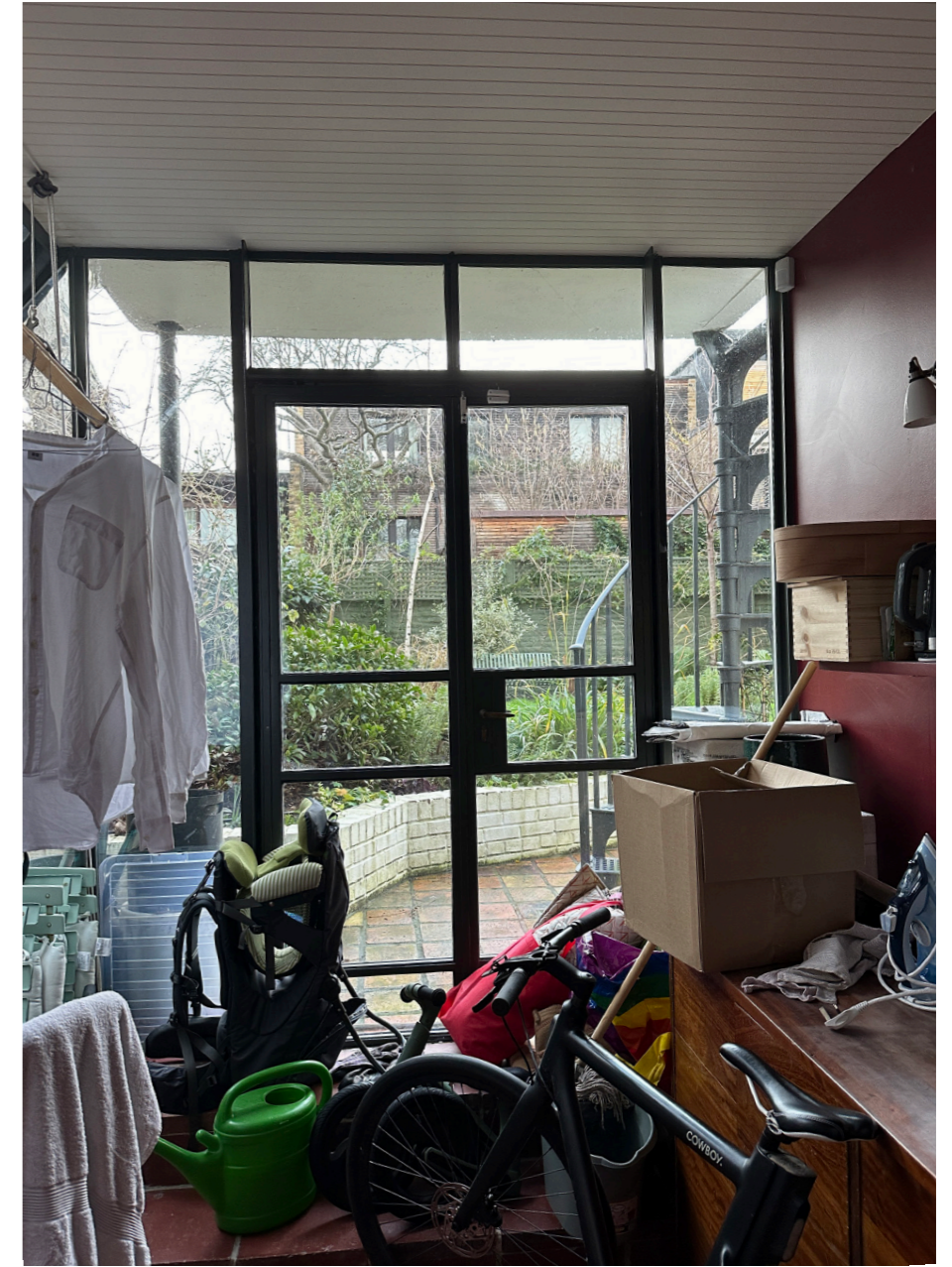
Fig 17. Existing rear glazed door from interior
