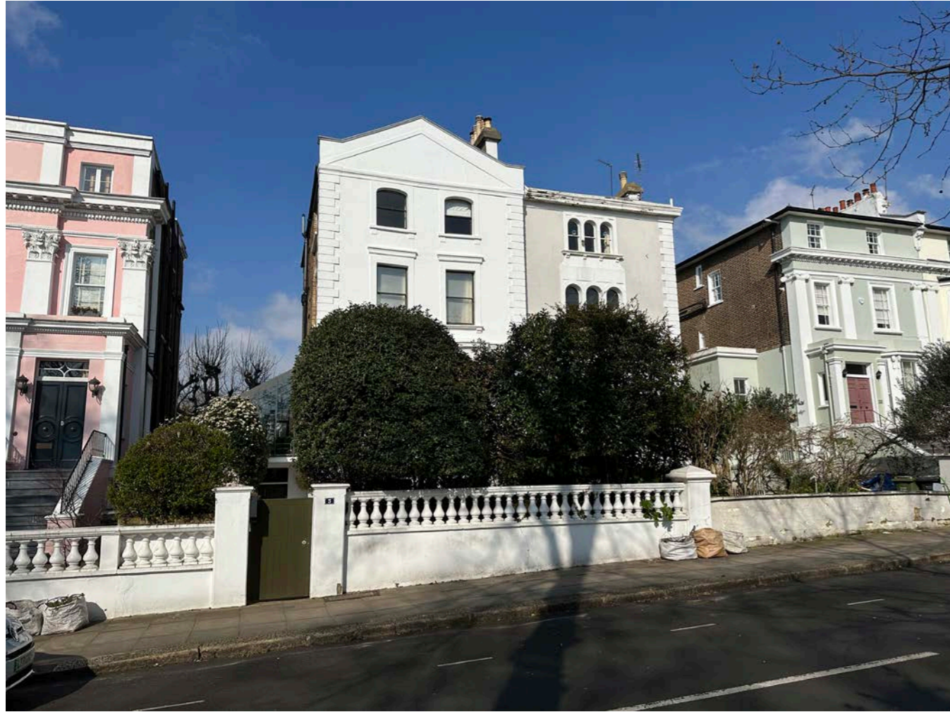
Fig 18. View from 3 Camden Square, North-East facing
