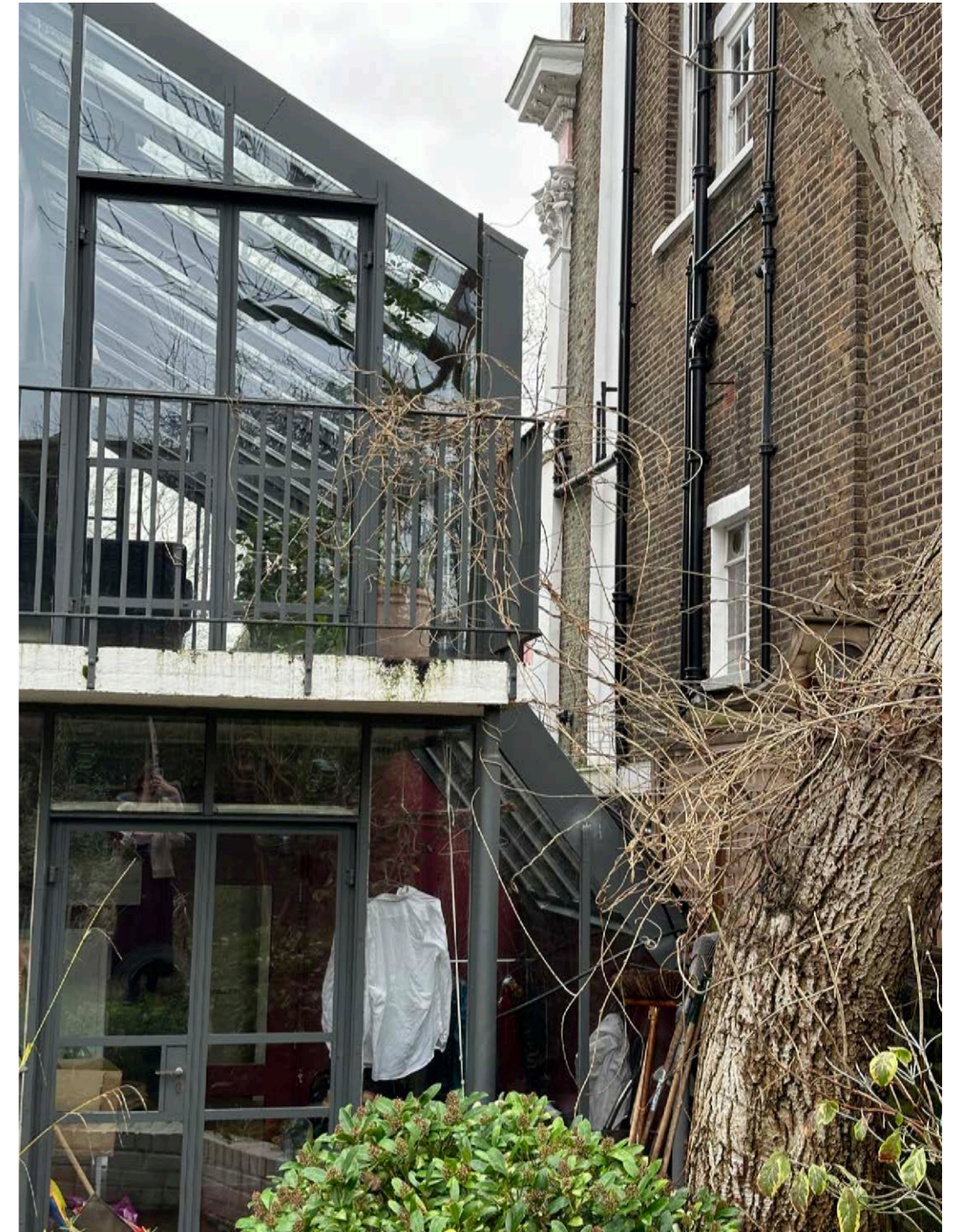
Fig 11. Rear elevation of existing extension
