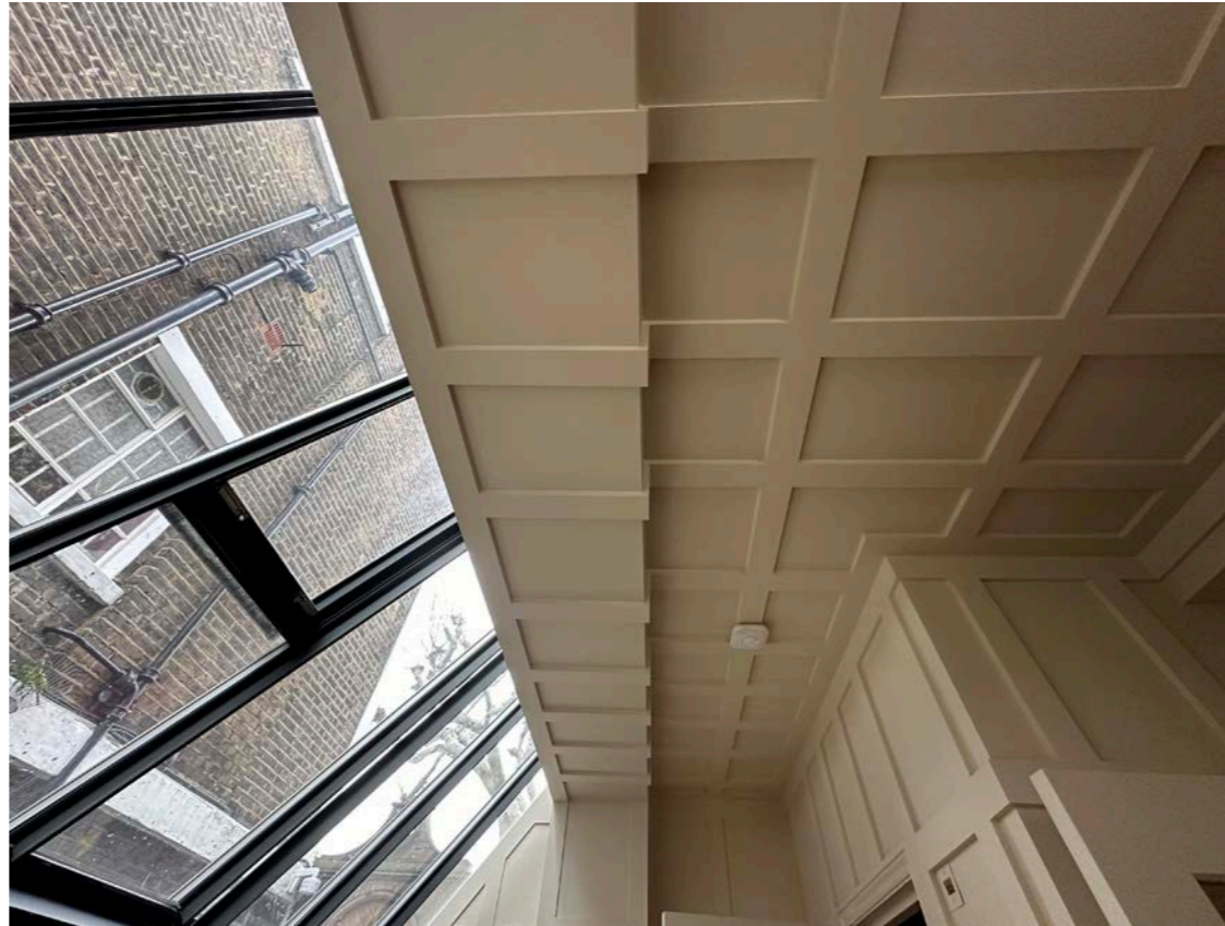
Fig 13. Existing glazing from inside front entrance
