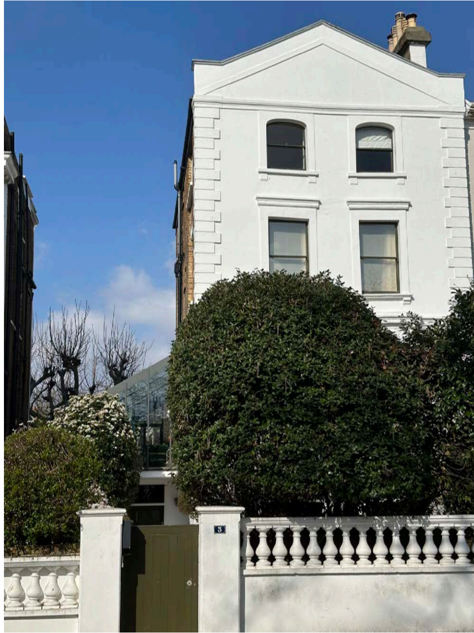
Fig 7. View of 3 Camden Square from street
