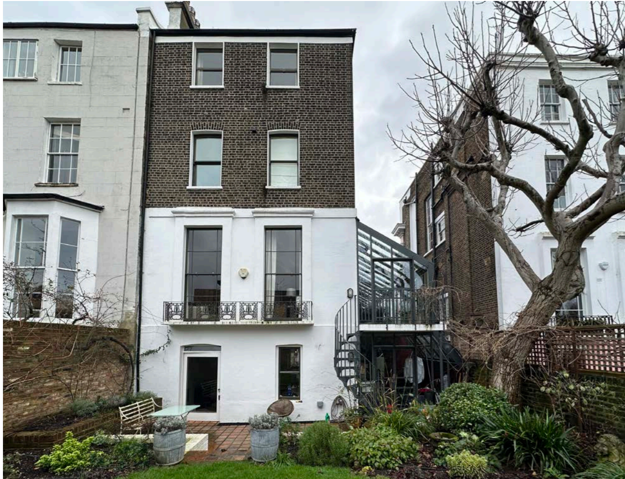
Fig 1. 3 Camden Square, Rear elevation
