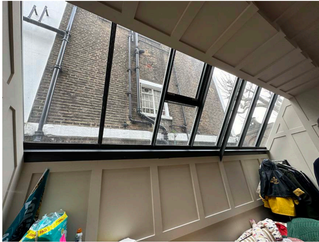
Fig 12. Existing glazing from inside front entrance
