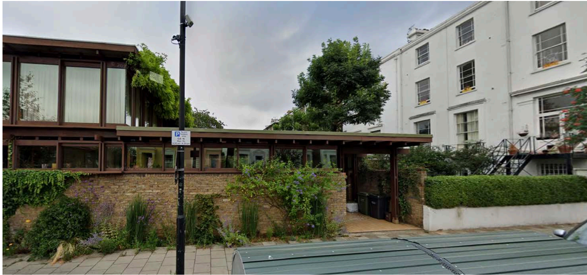
Fig 5. View to rear of Camden Square houses from Murray St
