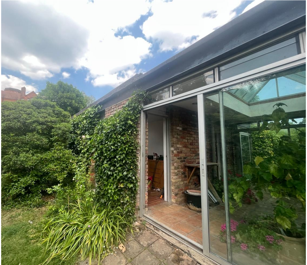
Photo showing perimeter steel arrangement over door openings
