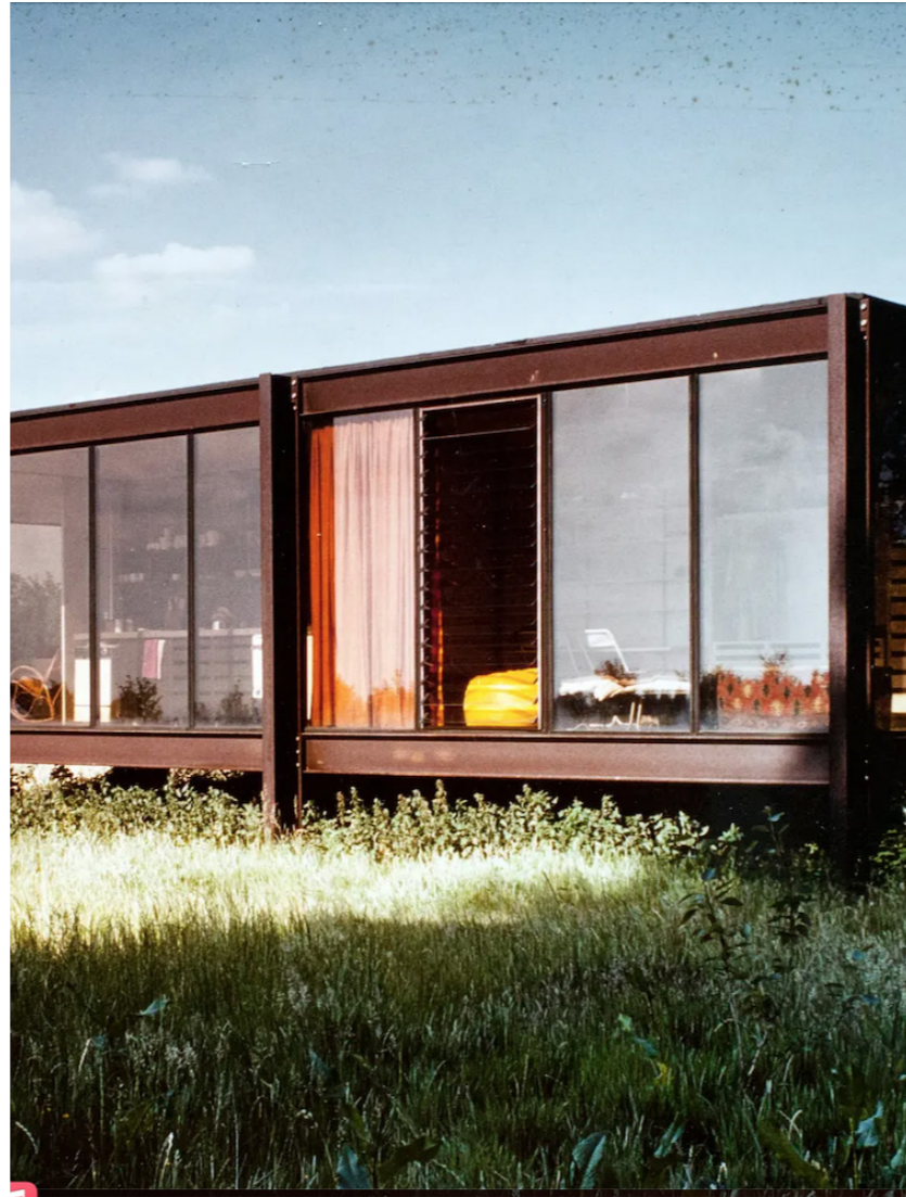
Georgie Walton's Fieldhouse's simple lightweight construction.
