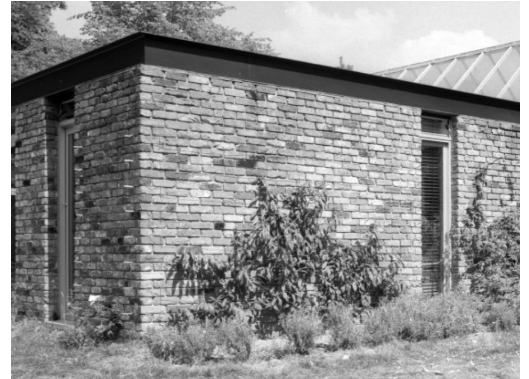
View showing original intention for roof detail and expressed steel.
