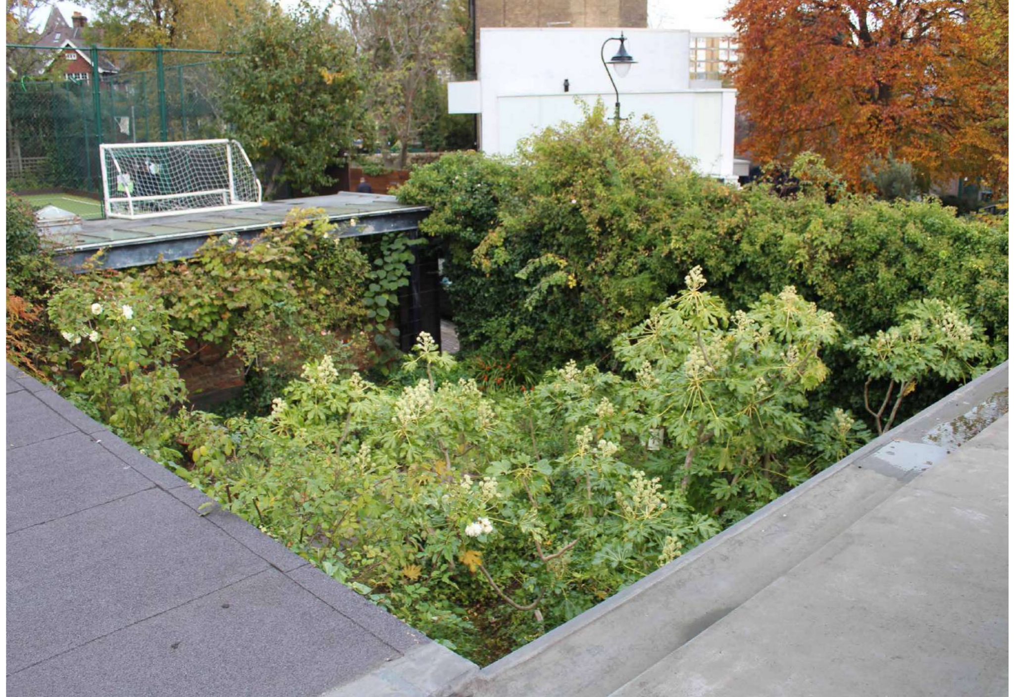
View from roof looking into the front Courtyard
