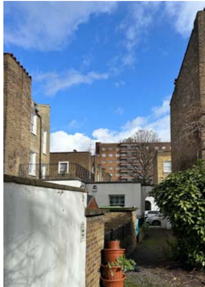
Figure 6.5 Existing view towards the rear of No. 26 Medburn Street along pathway from outside rear of No. 28 Medburn Street.
