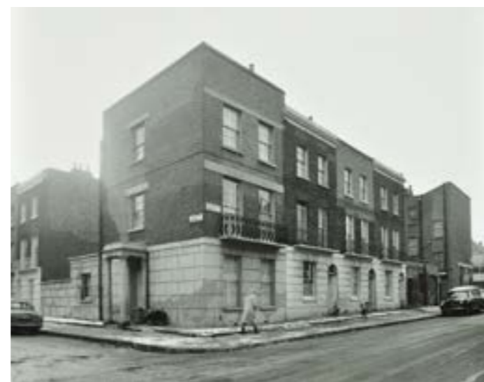
Figure 4.2 A comparative corner elevation from 1965 shows the difference in the lintel detailing Source: London Metropolitan Archives ©.
