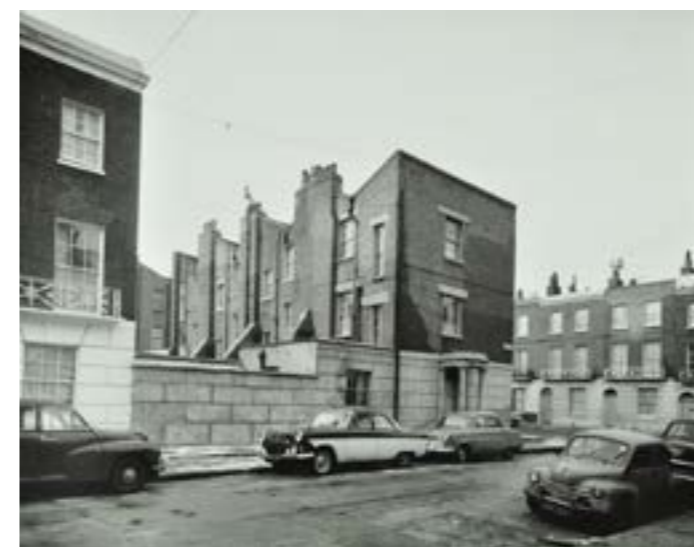
Figure 4.4 A comparative side elevation from 1965 shows the crude manner of the rusticated boundary wall and the earlier rear extension. There is also difference in the lintel detailing on the two upper floor windows Source: London Metropolitan Archives ©.
