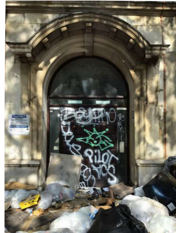
The right forecourt doors (right photo) are proposed to be replaced and repositioned at the same depth within the existing reveal as the existing doors to the left forecourt (left photo)
