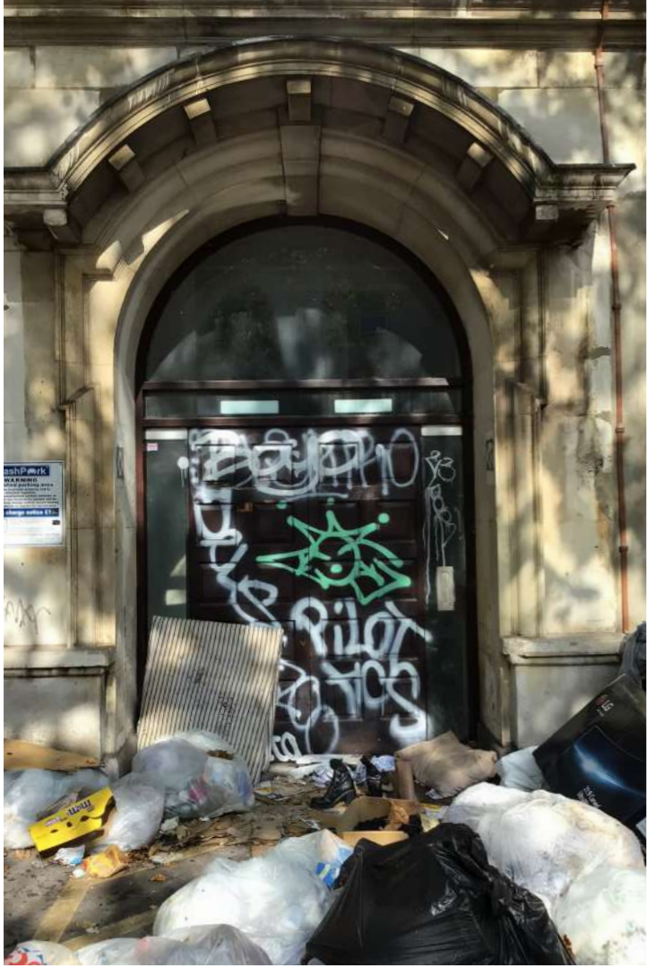
2. Existing doors proposed to be replaced
