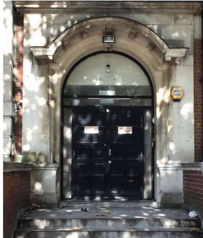
The right forecourt doors (right photo) are proposed to be replaced and repositioned at the same depth within the existing reveal as the existing doors to the left forecourt (left photo)
