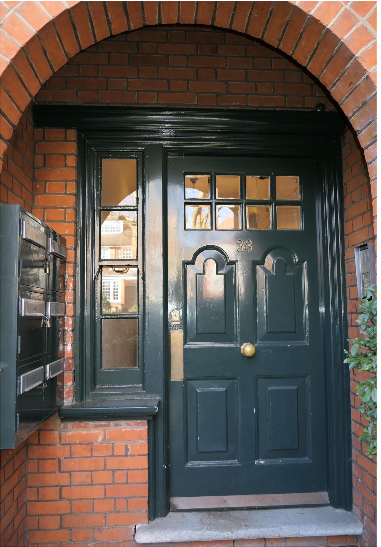
Photo 12: The front entrance, fitted with an intercom and mailboxes for each flat.
