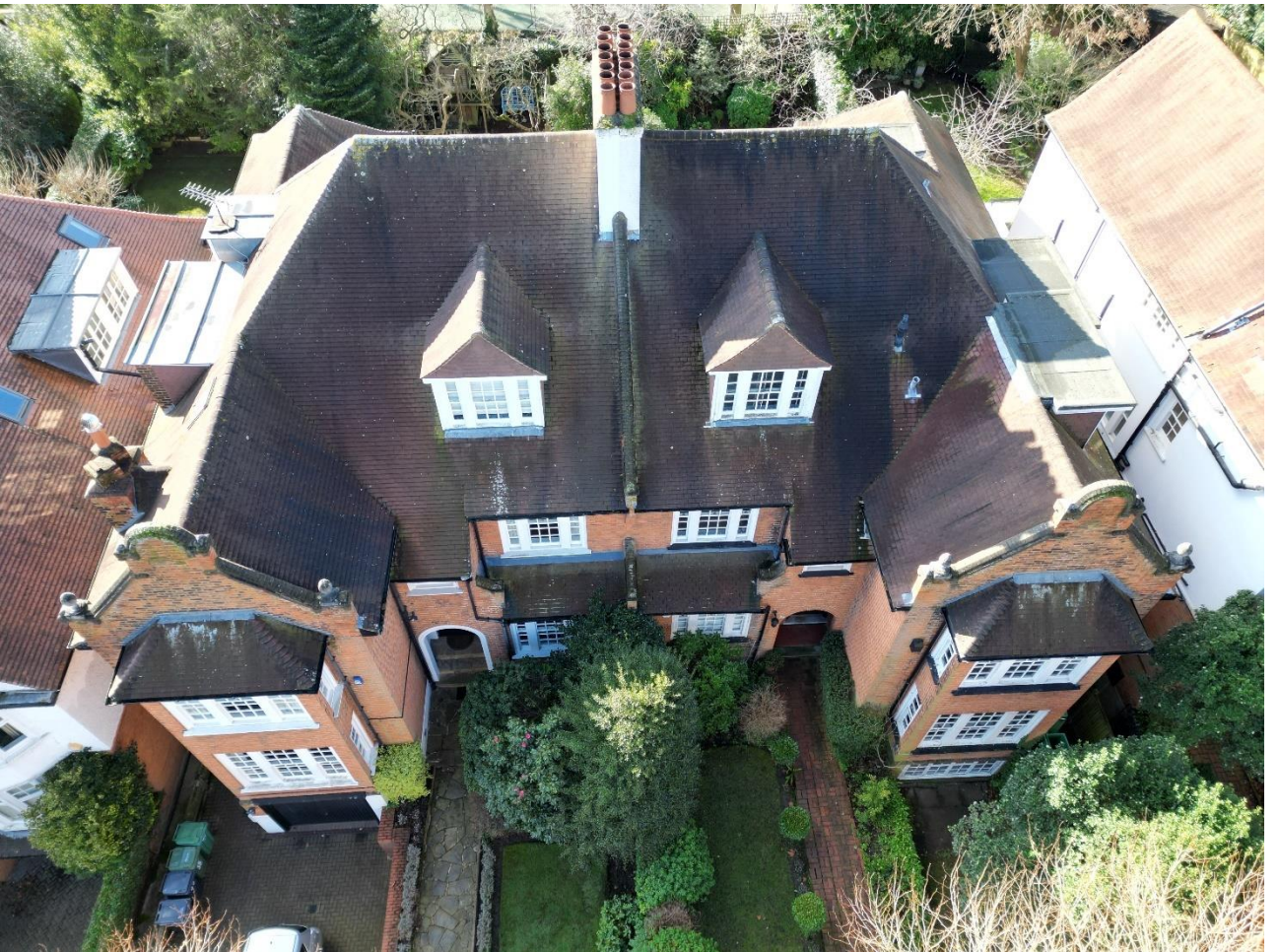
Photo 4: An aerial view of the front of 33 & 35 Ferncroft Avenue.
