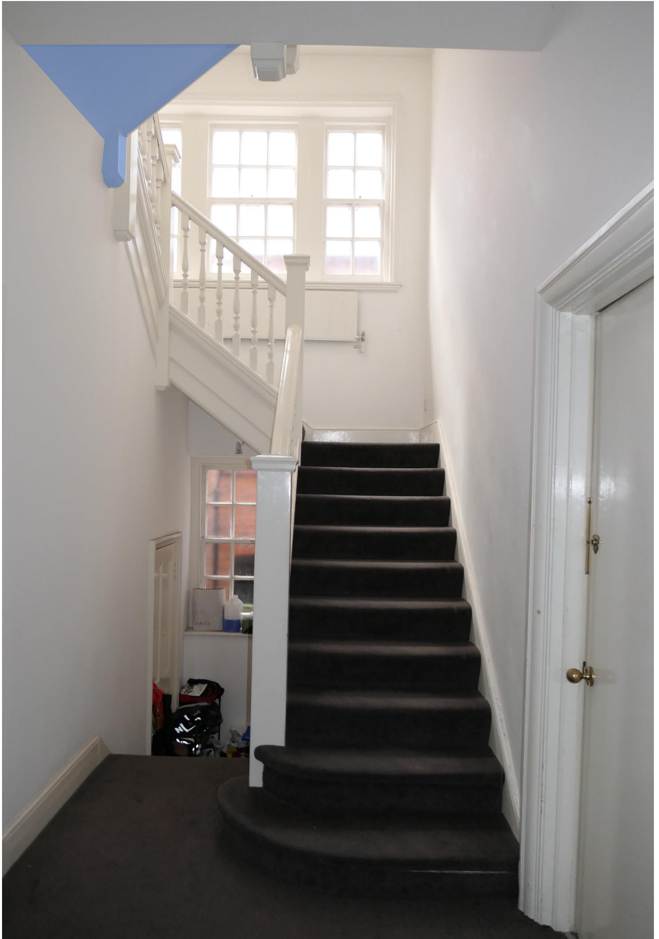
Photo 8: The ground floor stairwell, with the inserted flight above highlighted blue.
