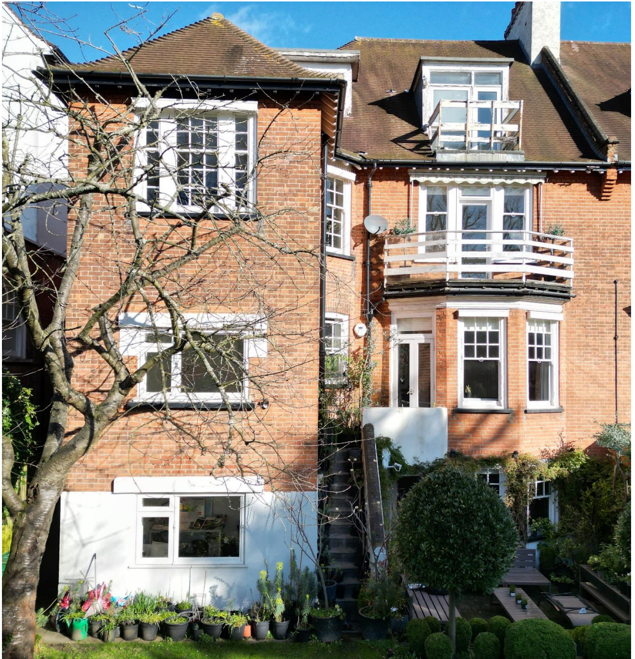
Photo 6: An elevated view of the rear elevation of 7 & 33 & 35 Ferncroft Avenue.
