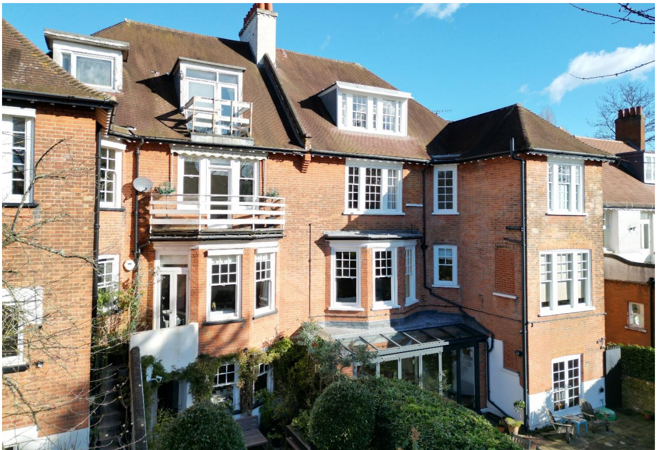
Photo 5: An elevated, oblique view of the rear elevations of 33 & 35 Ferncroft Avenue.
