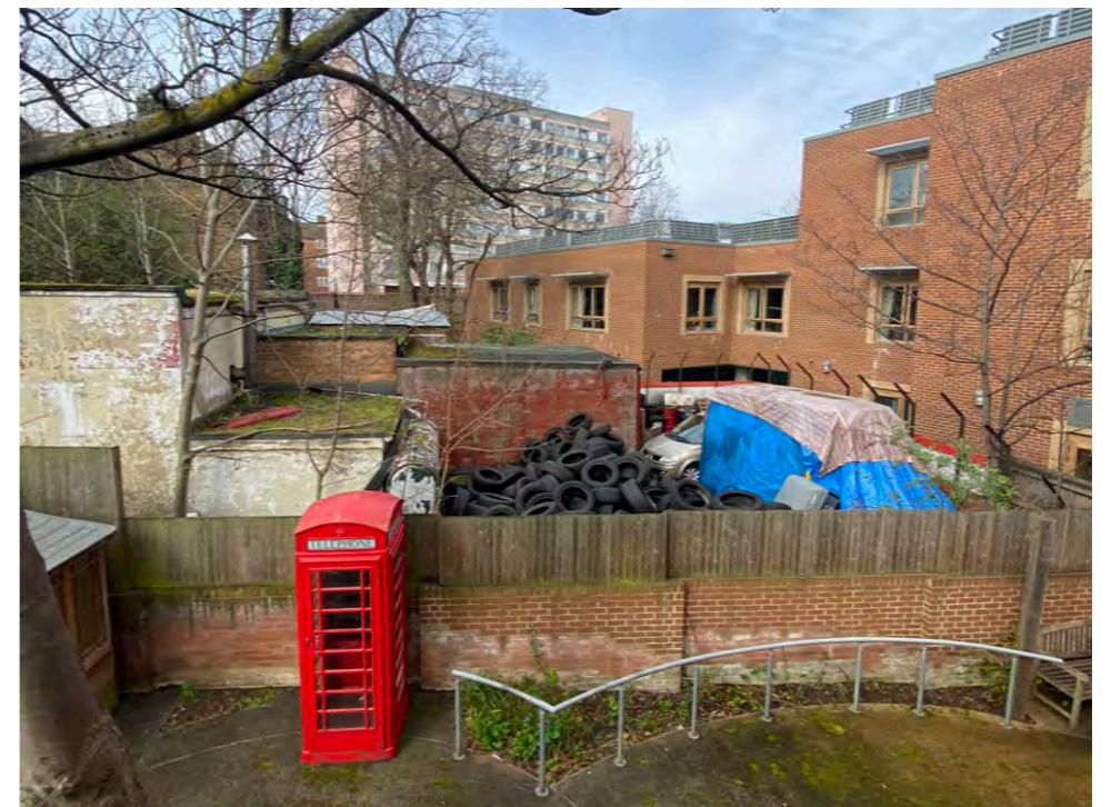
Back of service garage
