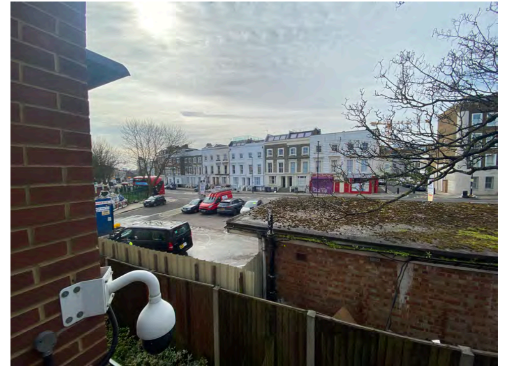
Roof of Reception block
