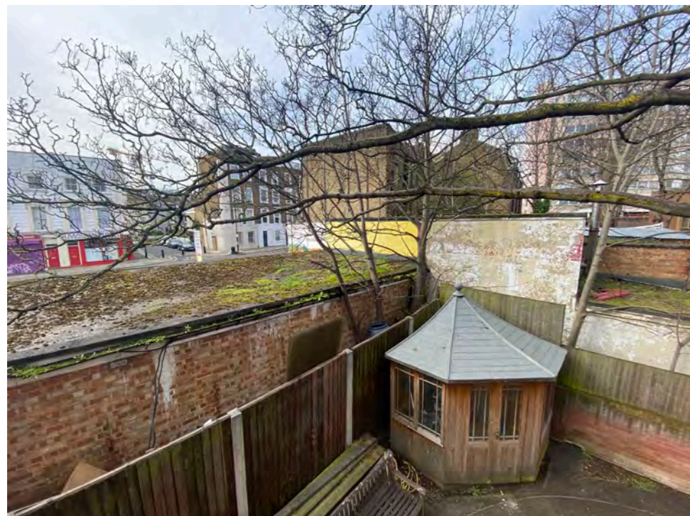
Roof of Reception block
