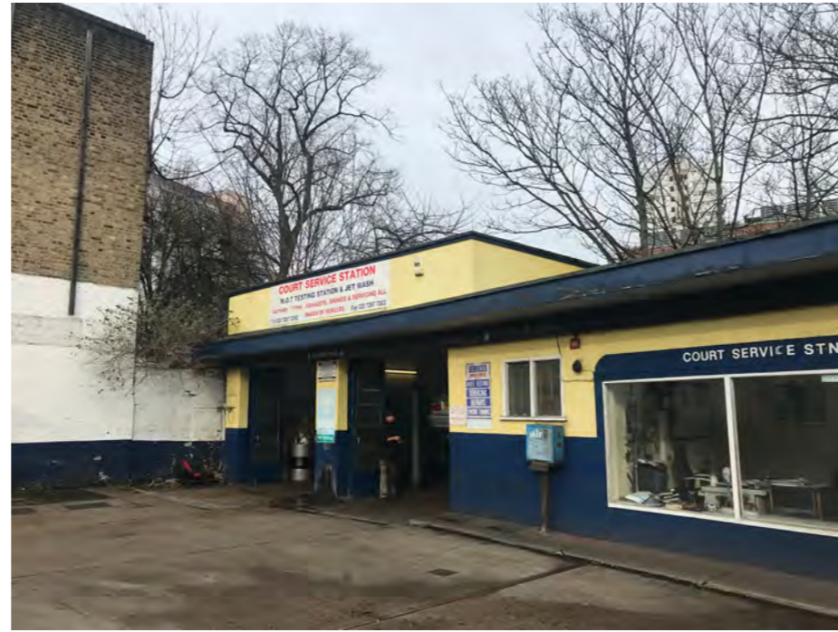
Malden Road - Context Garage
