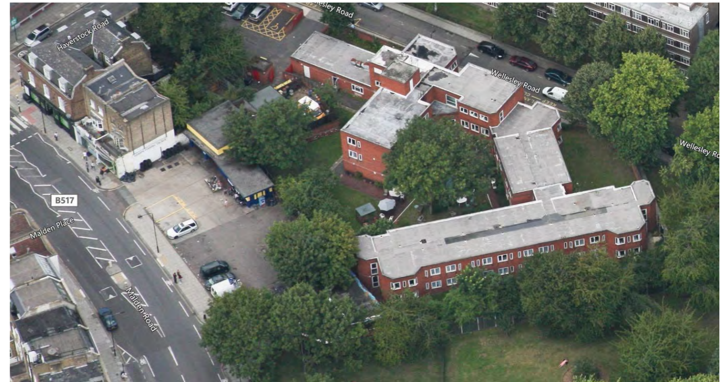
Care home building - South East view - Approx in year 2010
