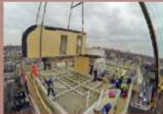
Module Delivery and Craning
