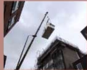
Module Delivery and Craning
