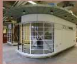
Modules Constructed in Factory Environment
