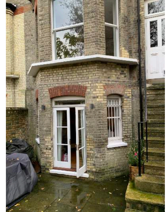
Existing Rear Lower Ground Floor Facade
