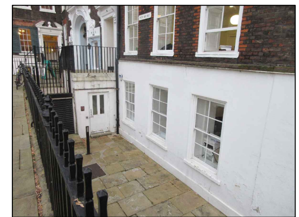
No 4 looking east.
