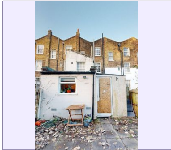
Existing Rear facade
