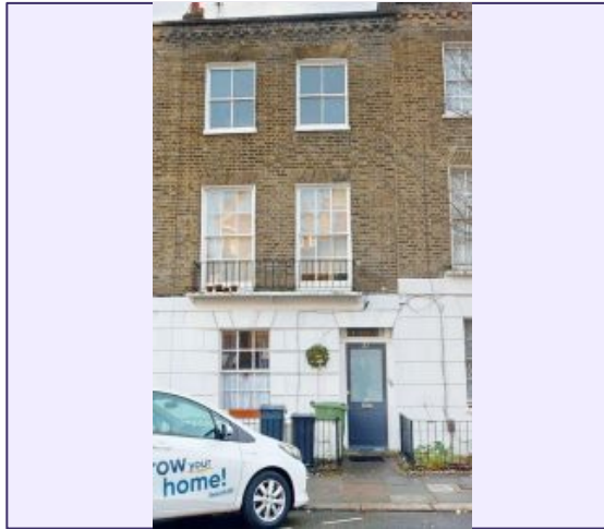
Existing Front facade
